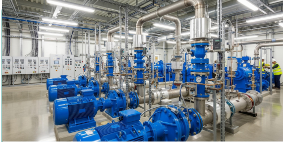
Chapter 3 Pumping Facilities
