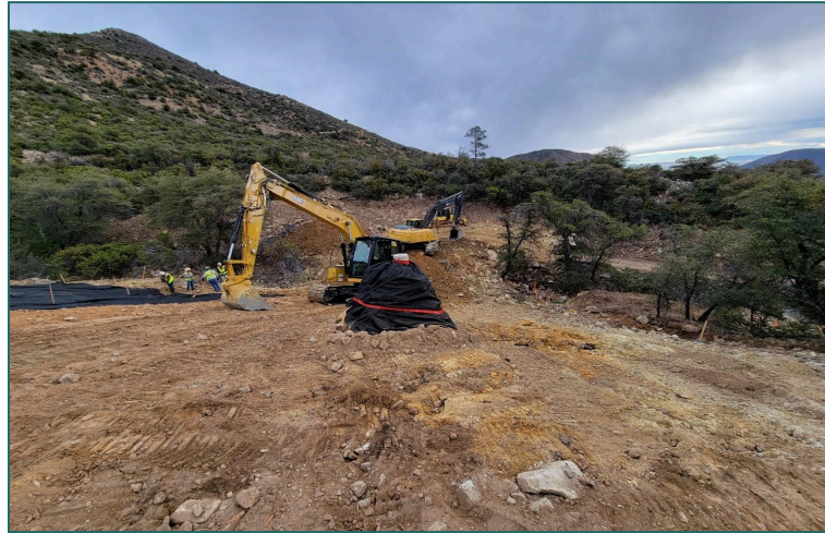
Construction of waste rock repository
