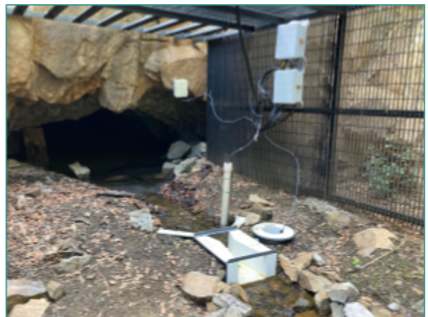
A mine adit at the historic Poland-Walker Tunnel continuously discharges into nearby Big Bug Creek, which is impaired for cadmium and zinc. Monitoring equipment at the mouth of the tunnel is capturing flow data, turbidity, and other parameters to help with the eventual remediation design.
