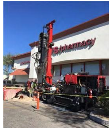
Drilling of Soil Vapor Monitoring Wells at CVS
