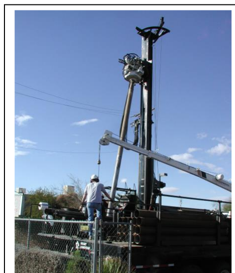
Monitor Well Installation
