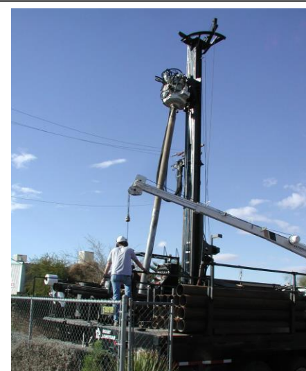
Monitor Well Installation
