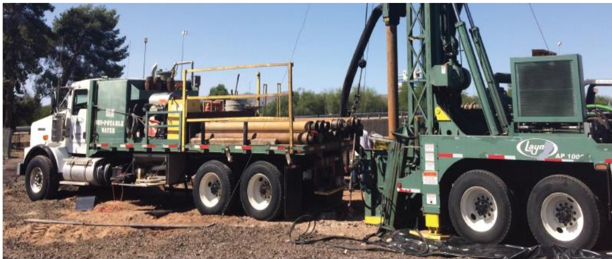
Groundwater monitoring well drilling and installation.
