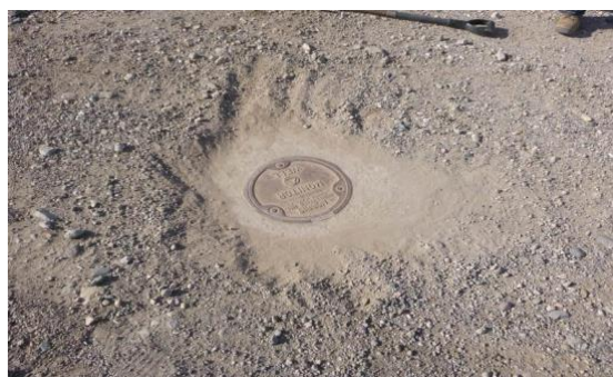
Groundwater Monitoring Well Vault
