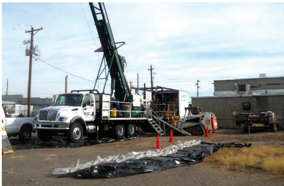
Figure 1 - Installation of soil vapor extraction wells at the North Plume.
