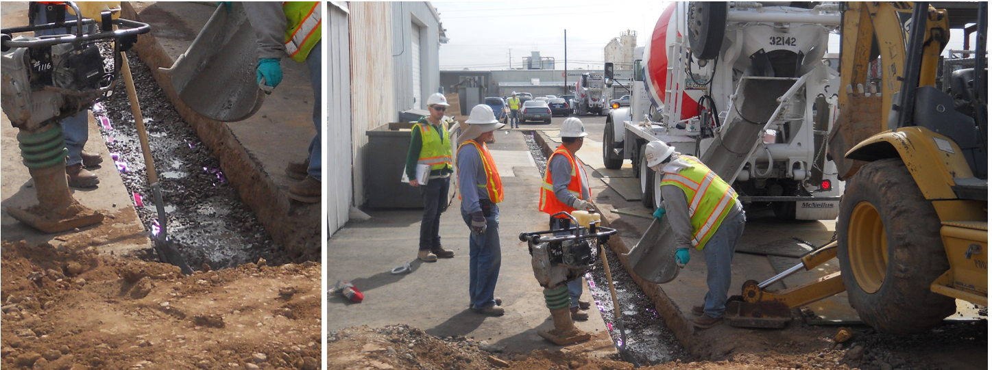
Figure 3 - Trenching and installation of groundwater treatment pumping lines at the North Plume.
