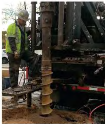
Drilling of Groundwater Well at 16th Street and Camelback Road
