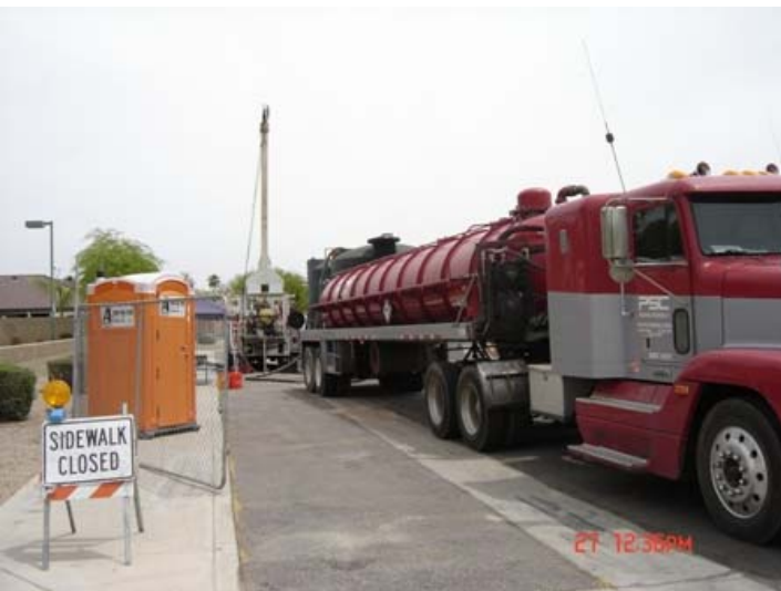
Pump rig for water removal
