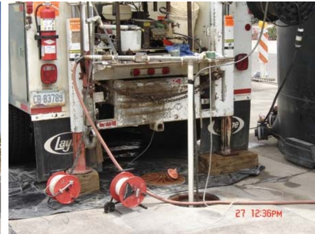
Pumping the new well
