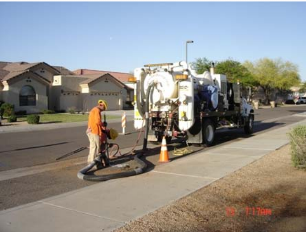
Air knifing the hole to 5 feet
