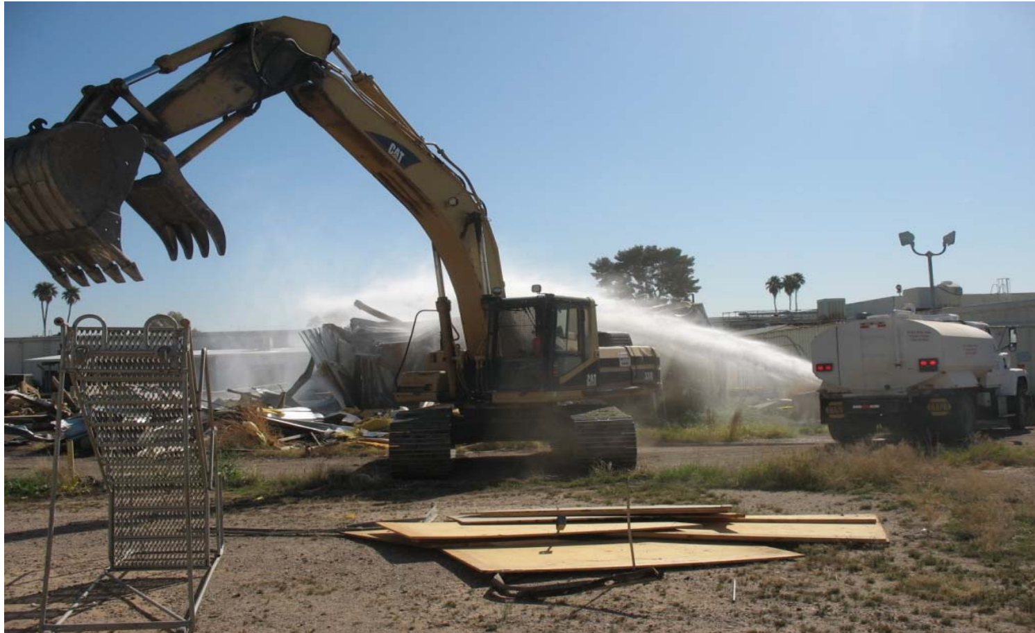
On-going Demolition with Dust Control Measures In Place
