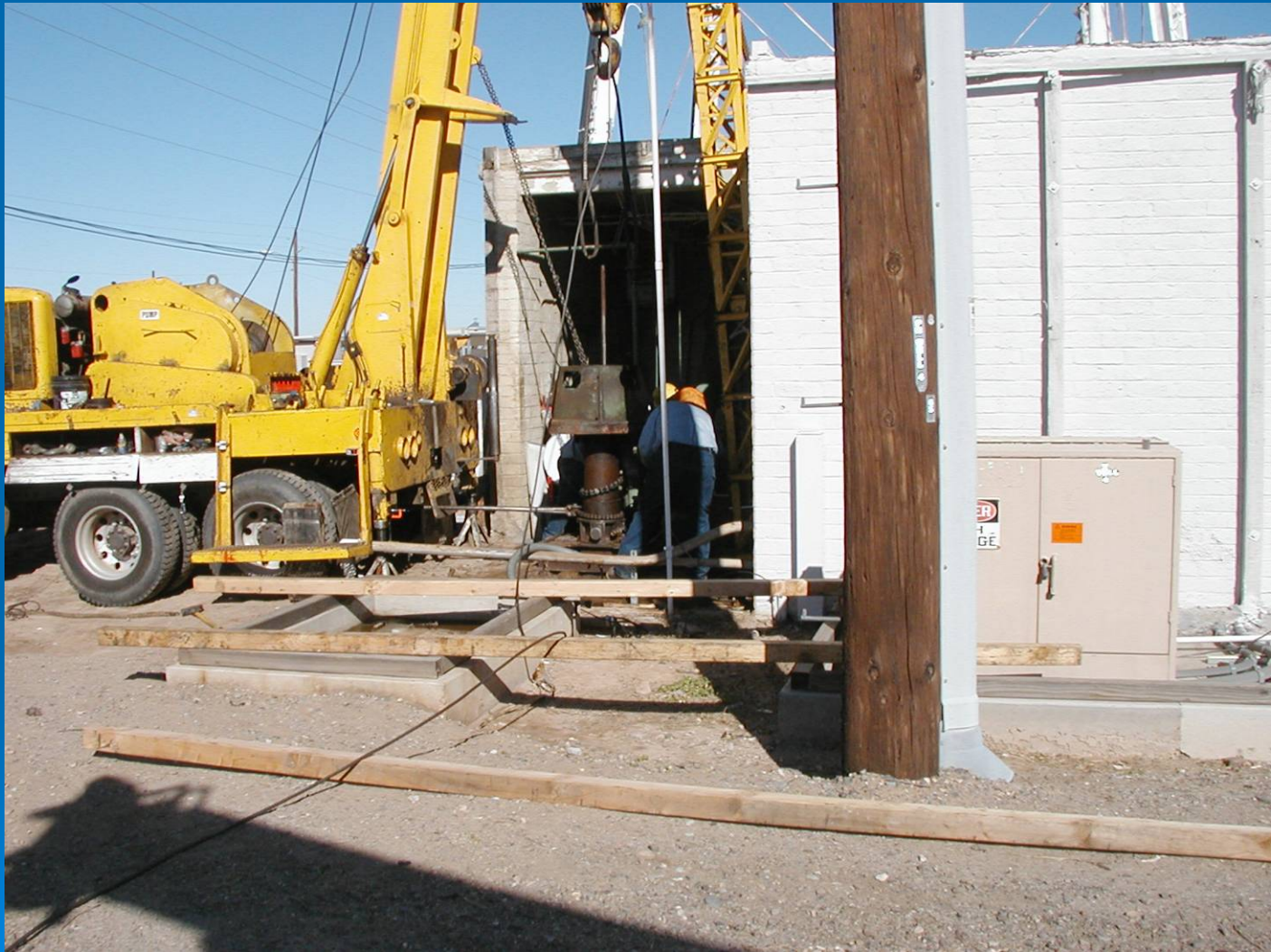
Removing Pump Column Pipe
