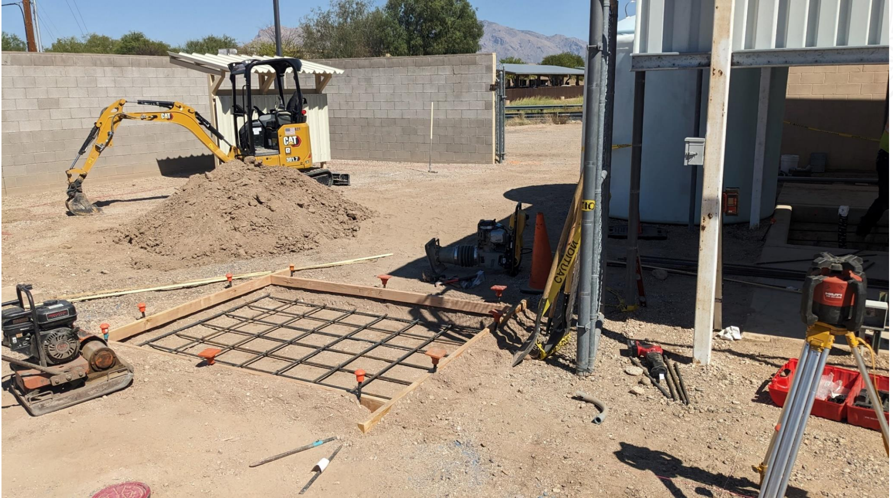
Ongoing treatment system upgrade
