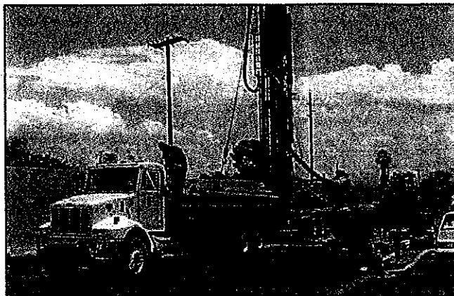
Drill rig installs a monitor well on a neighborhood street. Residents are notified prior to site work through an active community involvement program.
