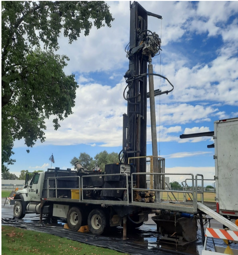
Drilling a groundwater monitoring well at the 51st Avenue and Camelback Road WQARF site
