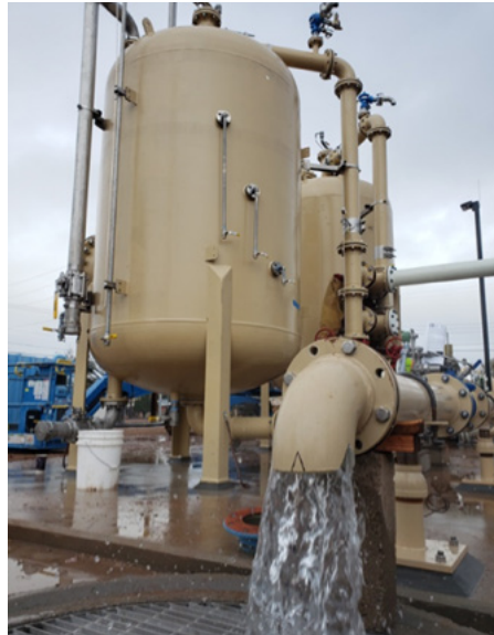
PFAS-free treated water being discharged from the Central Tucson PFAS Project Demonstration Treatment System.
