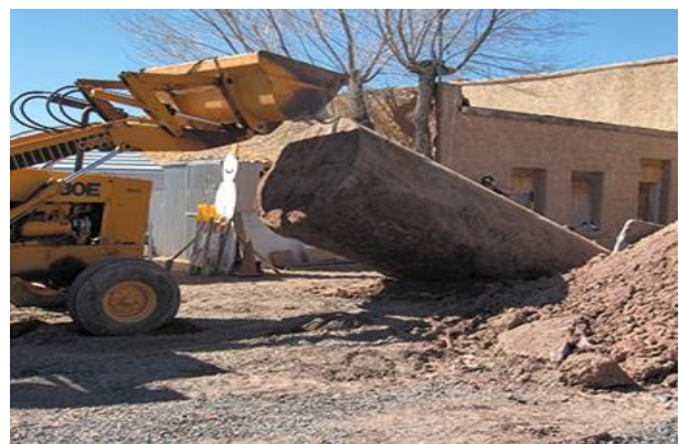
Underground Storage Tank removal J.J.'s Trading Post, Holbrook, AZ
