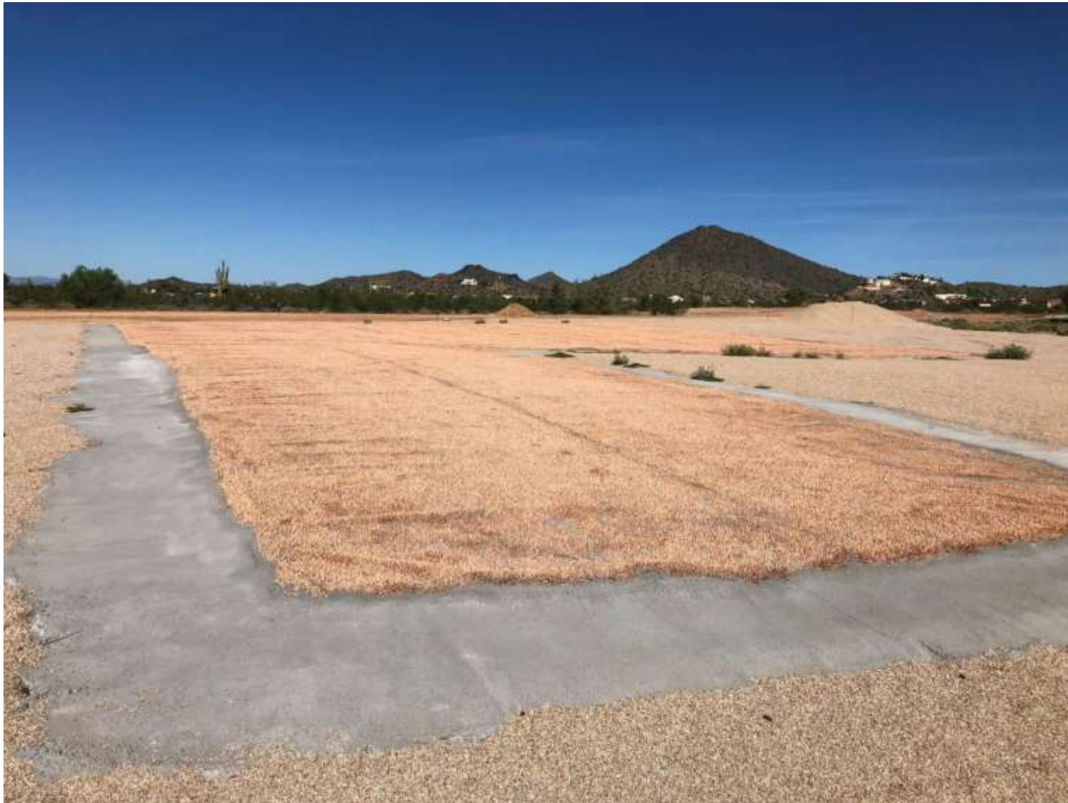
Figure 4 - SWMU 3, Engineered Cap (large cap) at New Burn Area
