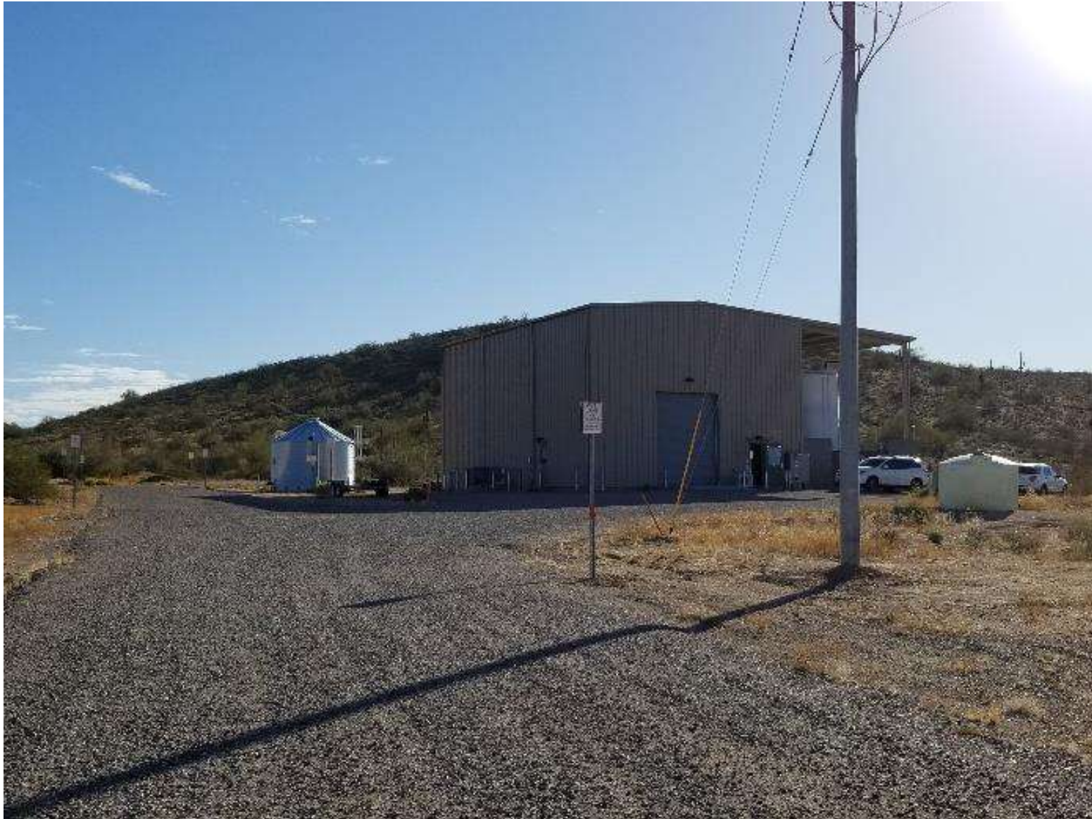
Figure 7- Groundwater Treatment Plant - Front
