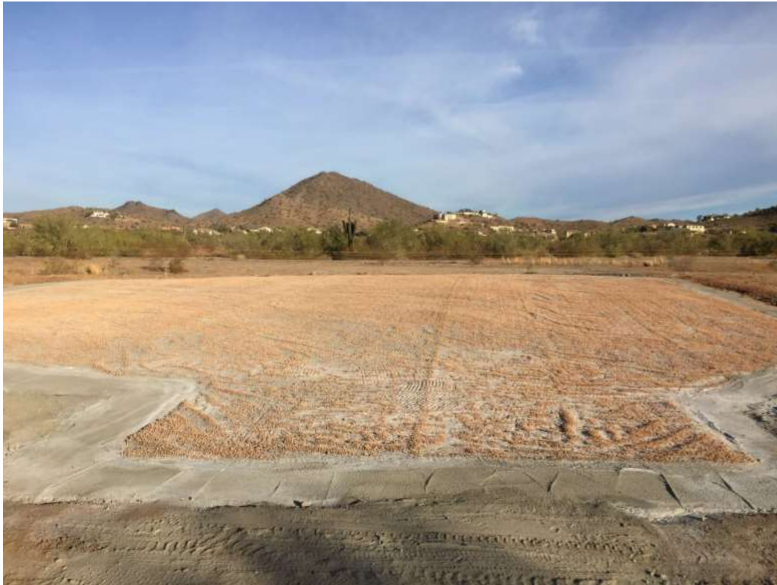
Figure 3 - SWMU 2, Engineered Cap at C-Complex Area
