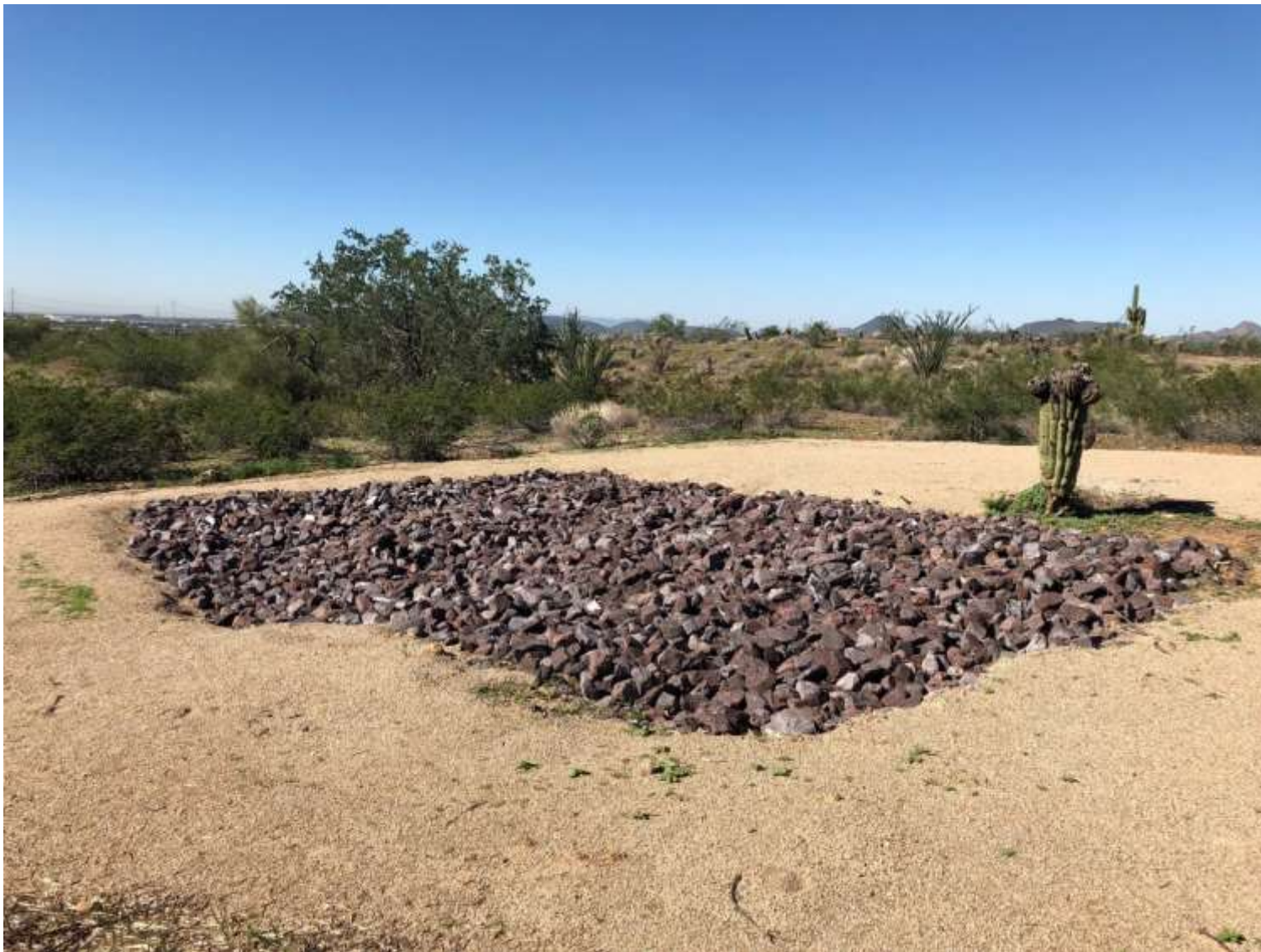
Figure 6- SWMU 5, Rip-Rap Cover at Old Burn Area
