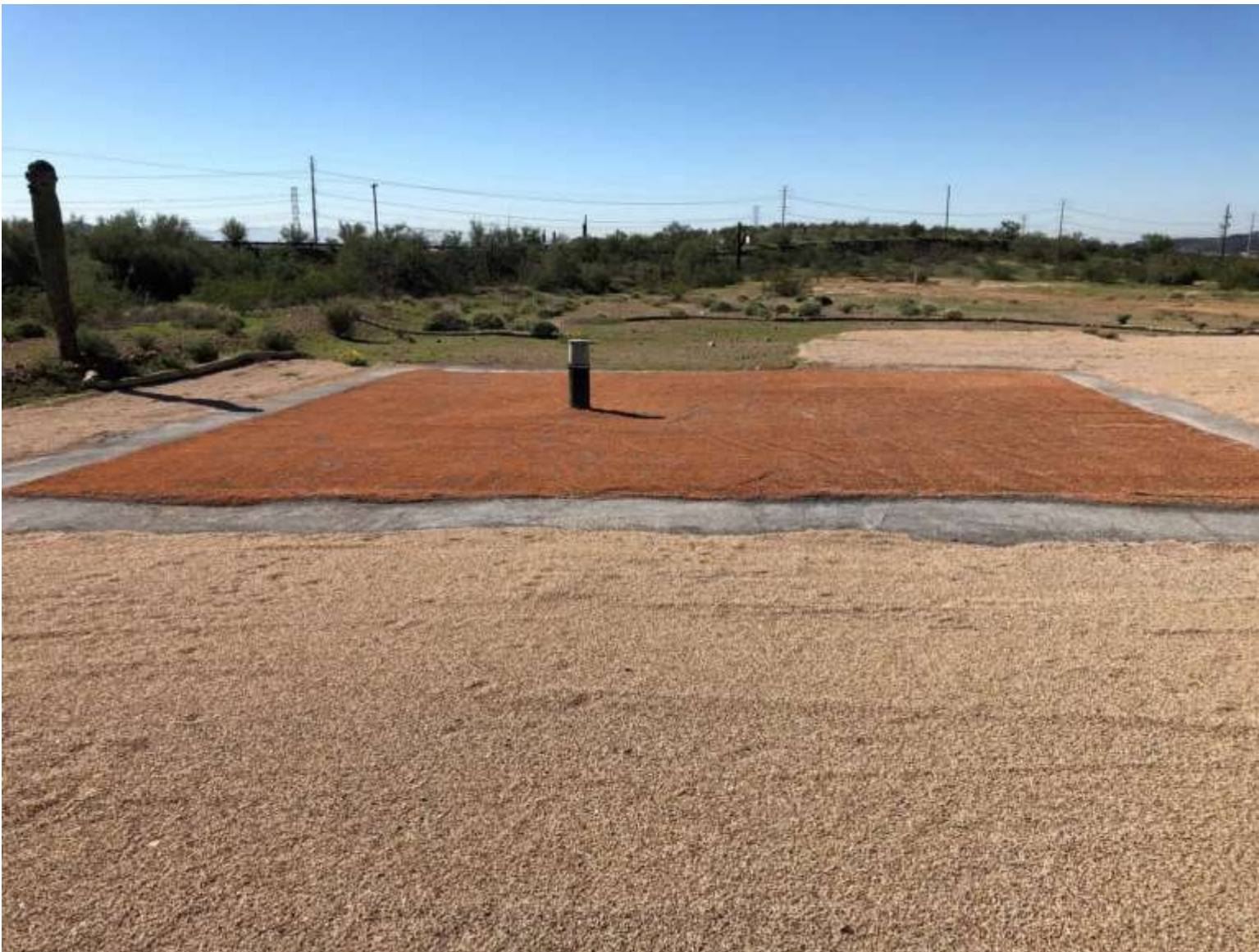
Figure 5- SWMU 4, Engineered Cap (Small Cap) at New Burn Area)
