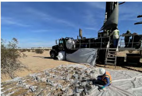
Fieldwork at IR Site 9 includes installation of a groundwater monitoring well
