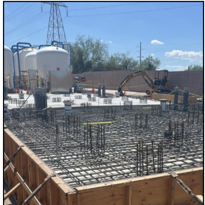
Figure 3: IX System construction in progress
