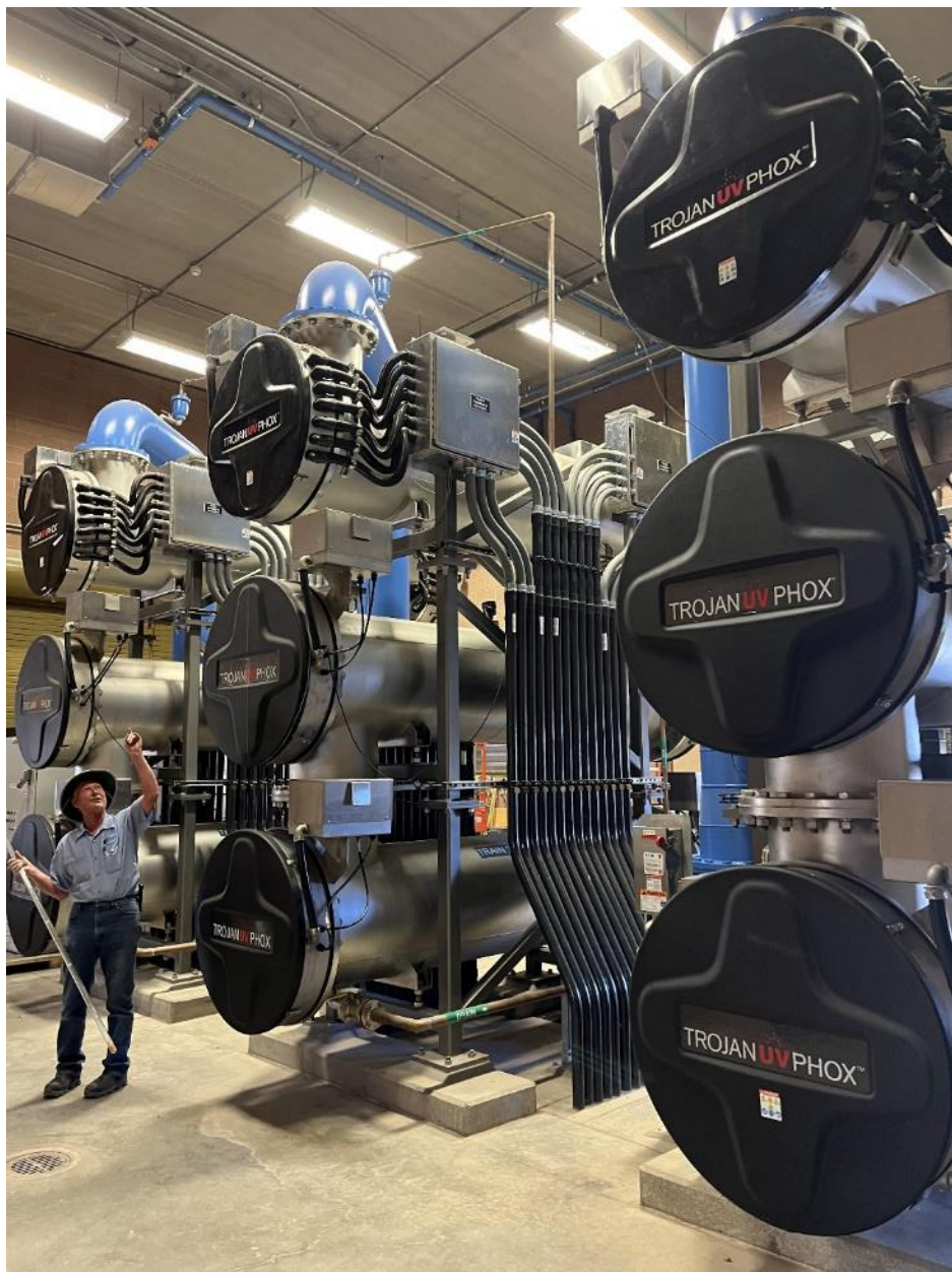
Figure 27- TARP UV PHOX system
