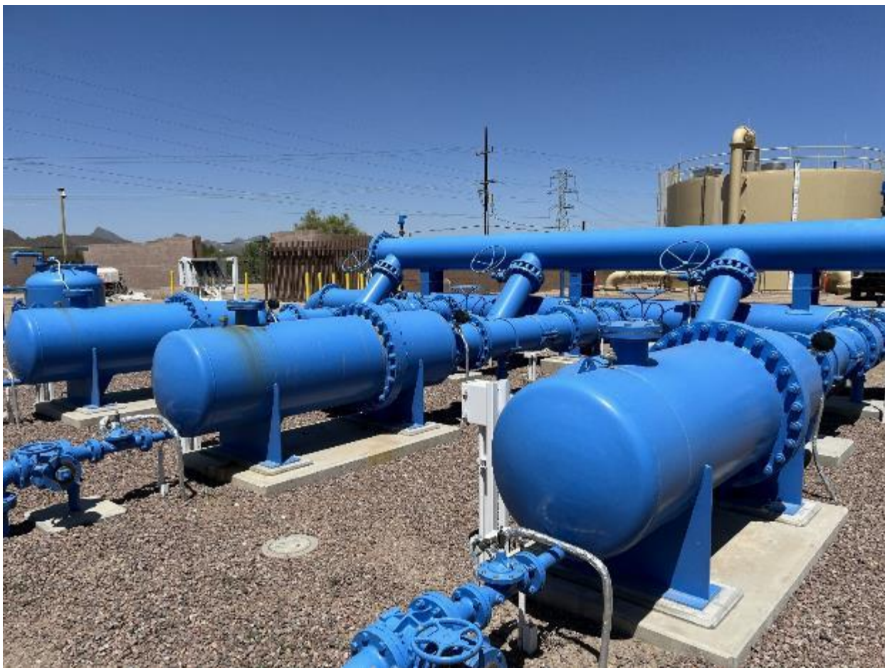
Figure 20- TARP Desanding Hydrocyclones
