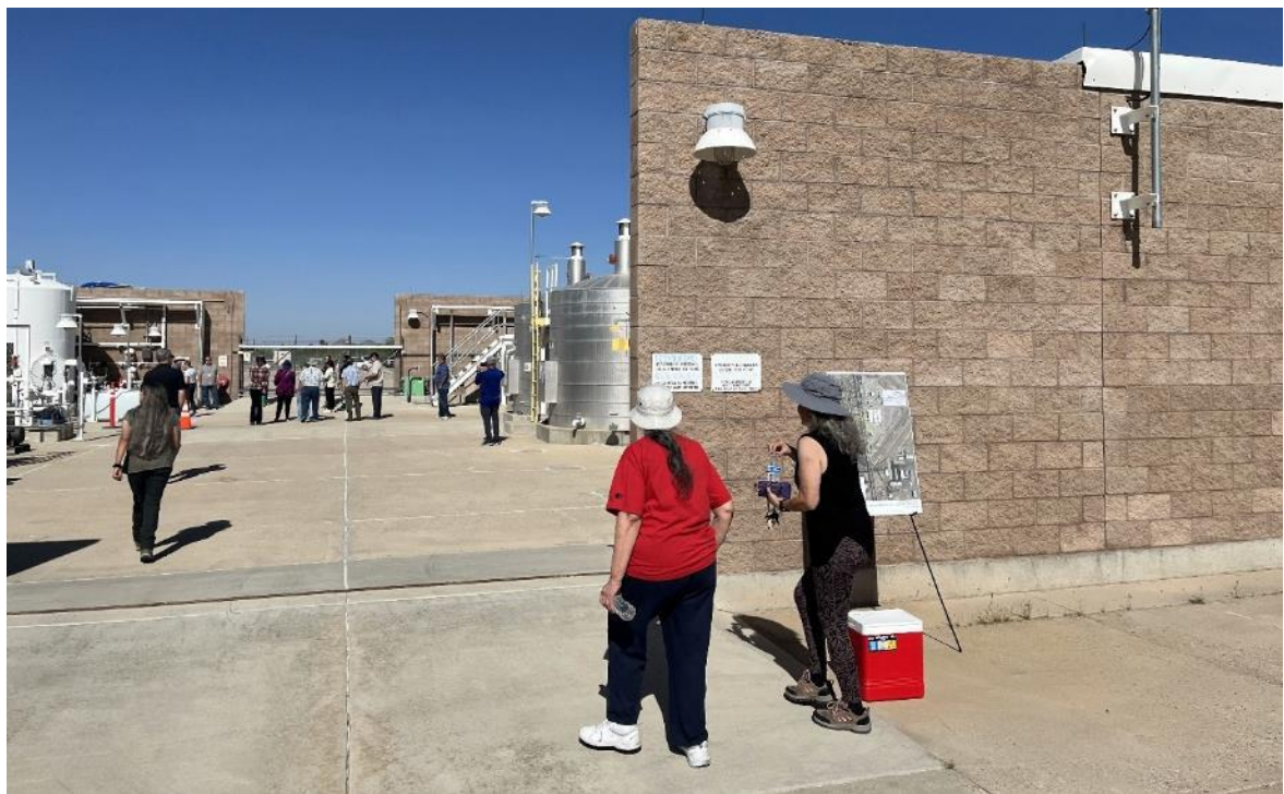
Figure 1- Entrance to Airport Properties GWTP
