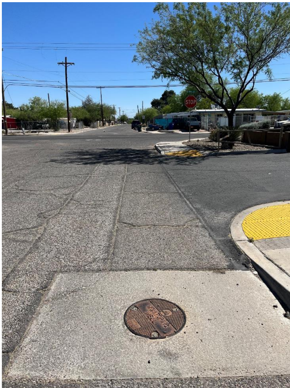
Figure 39- West Plume B flush mount well
