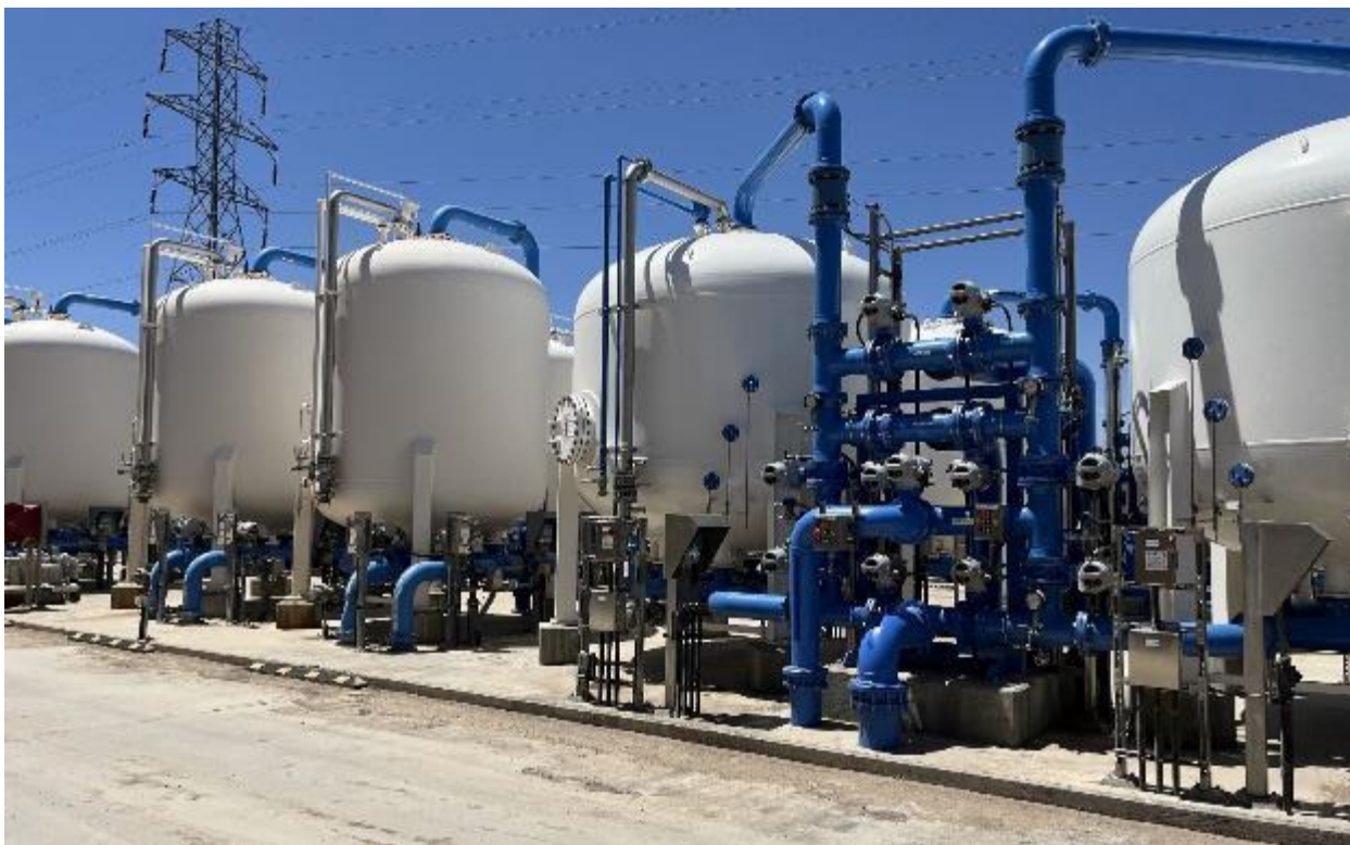
Figure 28- TARP GAC vessels (900 gpm on right)
