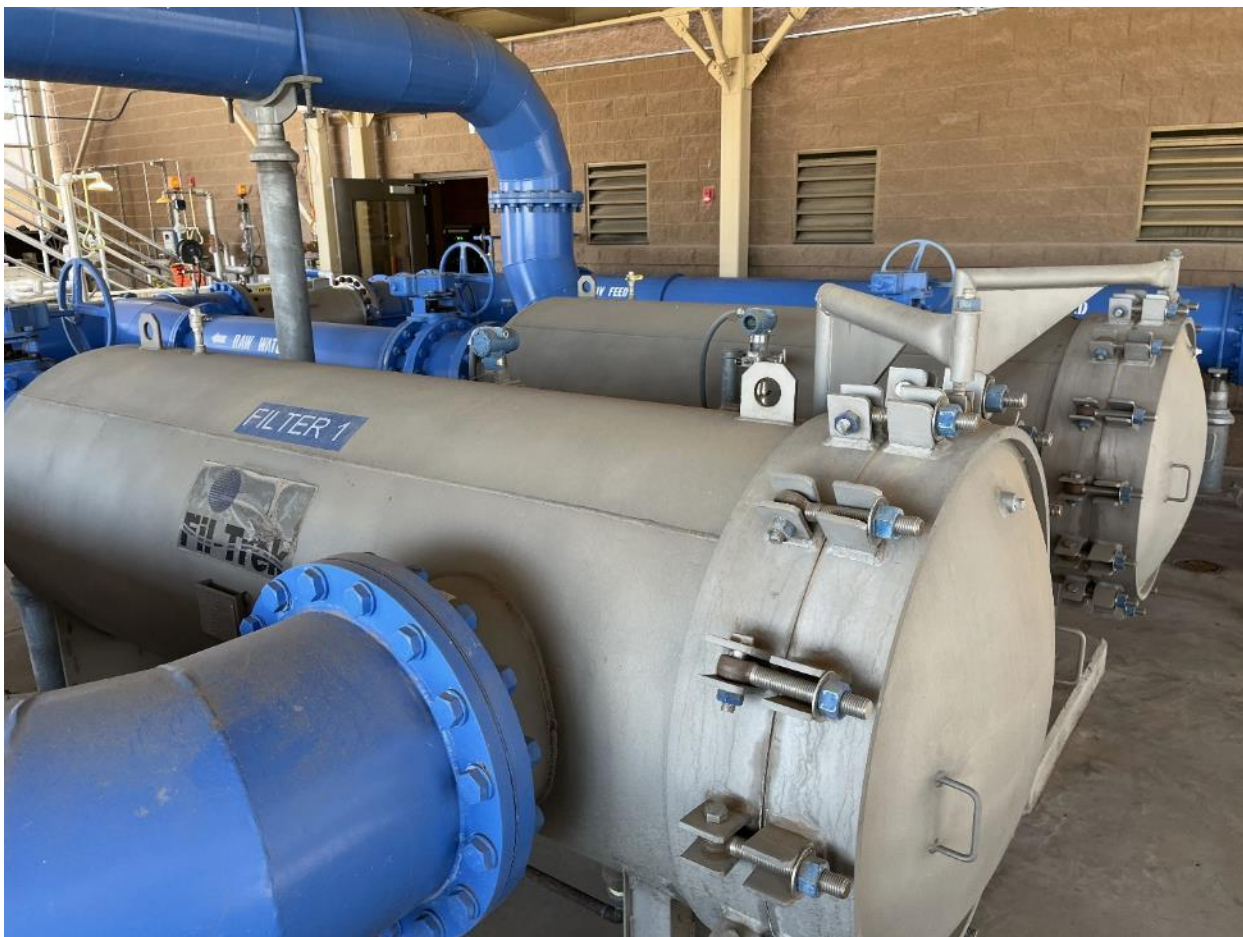
Figure 22- TARP silt cartridge filters
