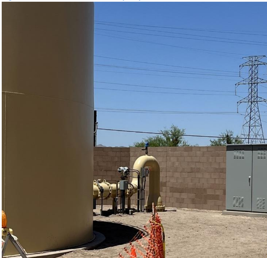
Figure 31- discharge point to river
