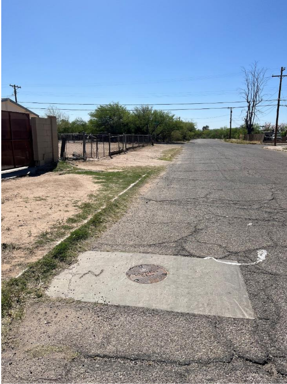
Figure 40- West Plume B flush mount well
