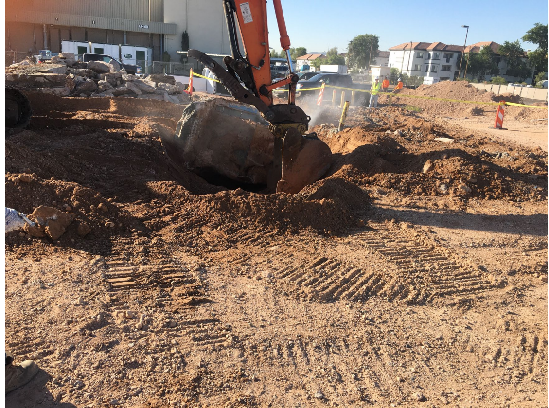
Sump (intact) being removed
