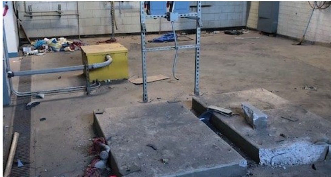
Photo 2 SVE system removed from AD building, only concrete slabs remain.
