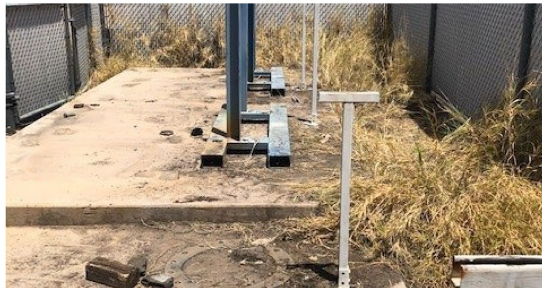
Photo 13 View of four carbon vessels removed from former location.
