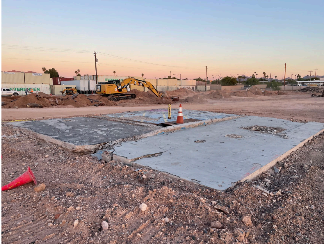
Remaining slab and sump prior to excavation
