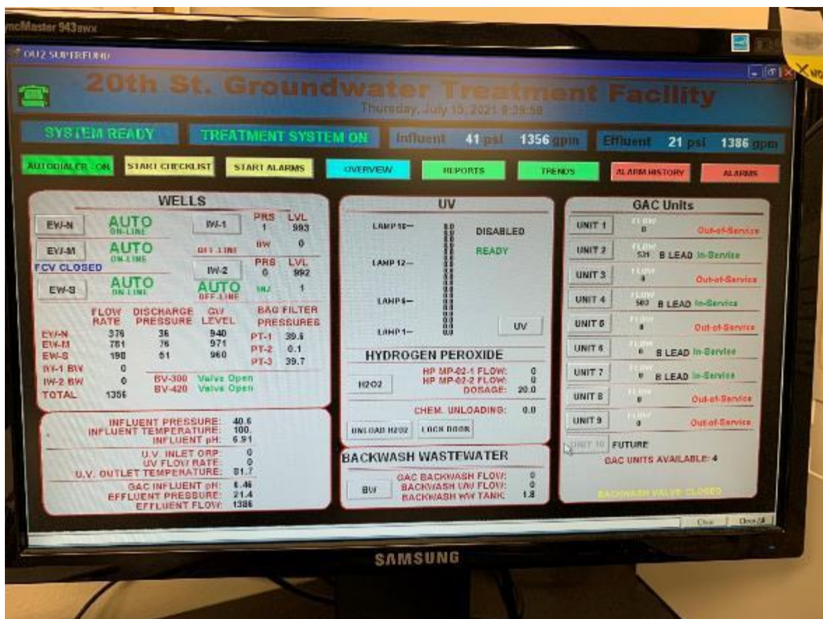
Figure 14- OU2 Treatment Facility control console
