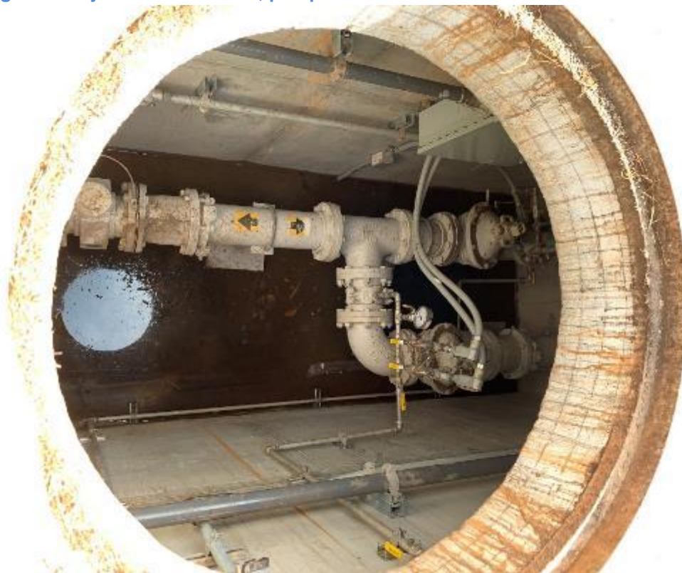
Figure 25-Injection well 2 vault, pump removed
