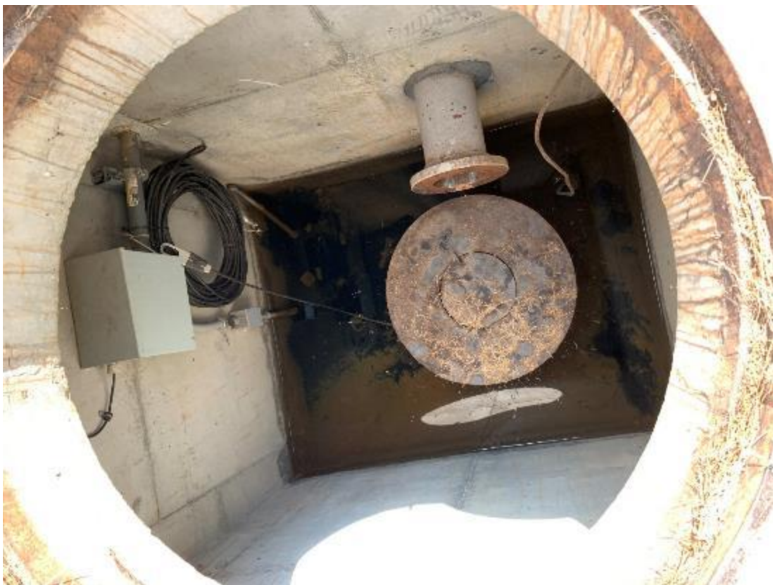
Figure 25-Injection well 2 vault, pump removed
