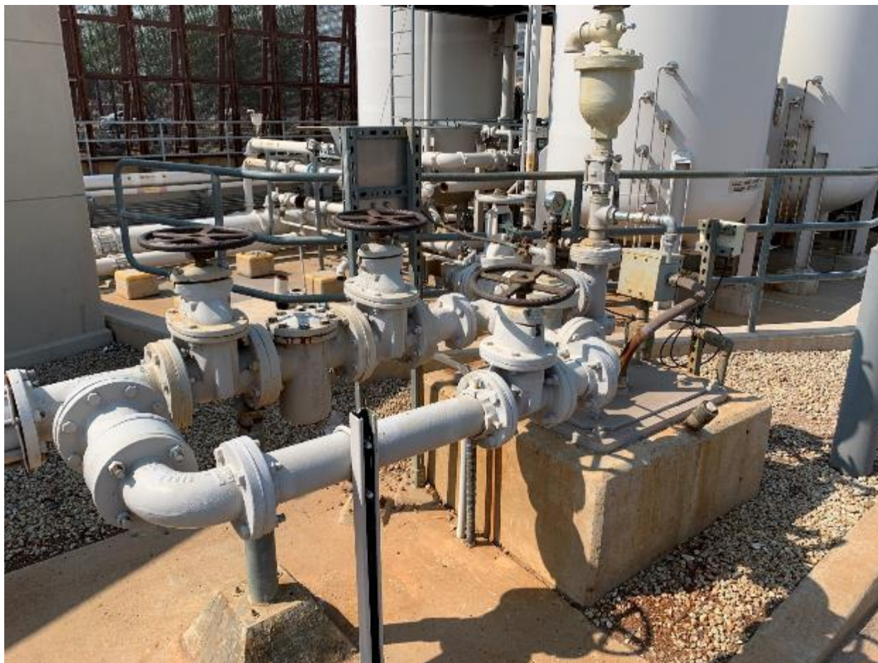
Figure 22-OU2 South extraction well with sand filter
