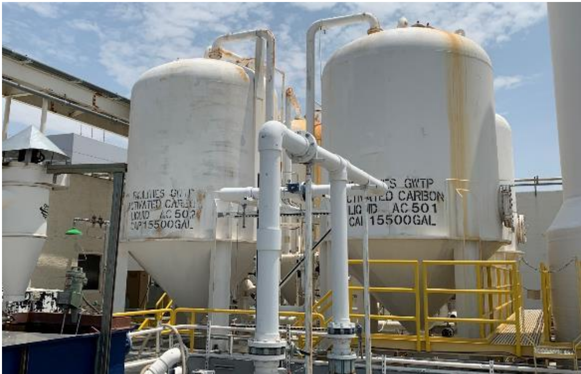
Figure 34- OU1 Liquid GAC vessels
