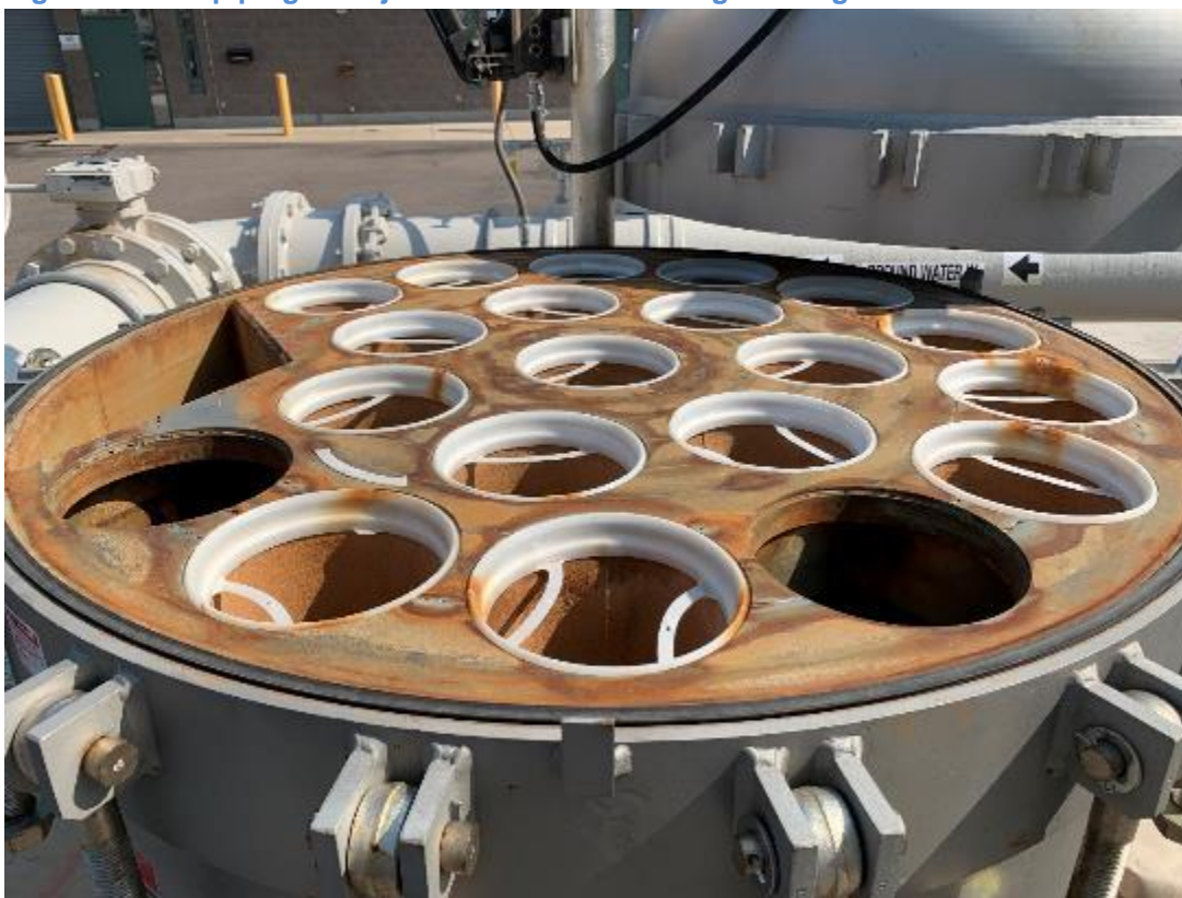
Figure 17-OU2 injection well bag filter interior, showing corrosion to be milled off
