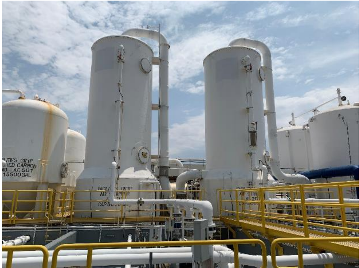
Figure 33- OU1 Air stripper towers
