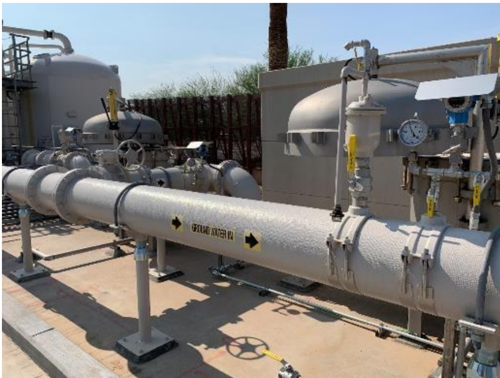
Figure 16-OU2 piping for injection well backwashing and bag filters
