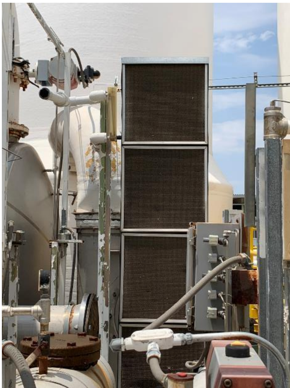
Figure 36-OU1 Filter box for air intake
