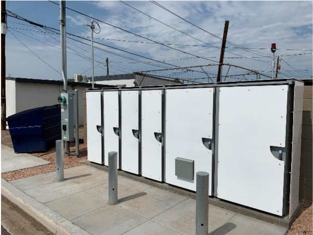
Figure 27-Electronics cabinets for injection wells
