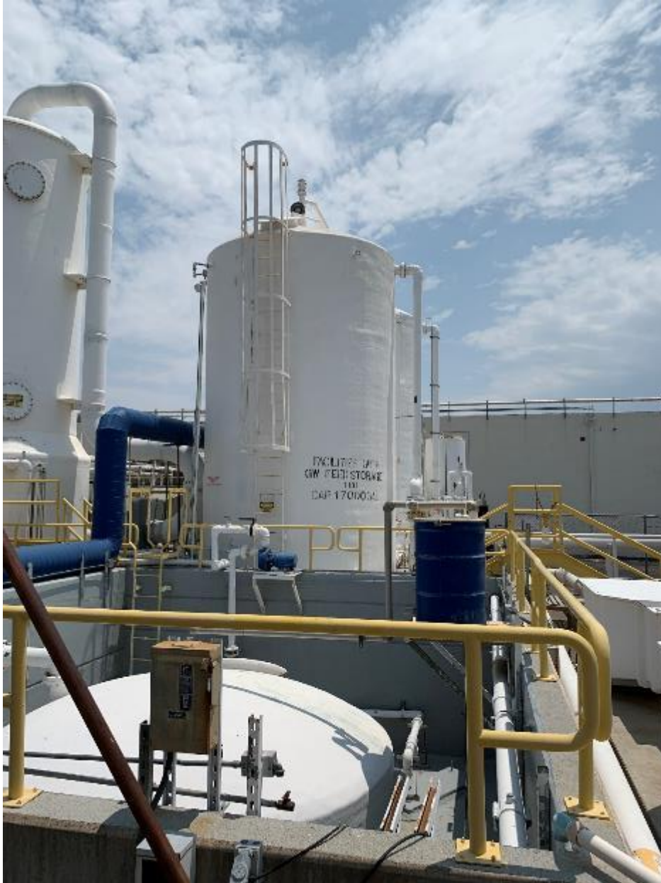
Figure 32-OU1 Feed storage tank
