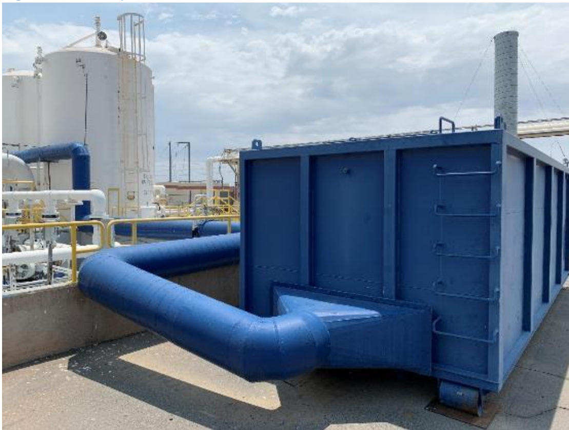
Figure 35- OU1 VGAC vessel
