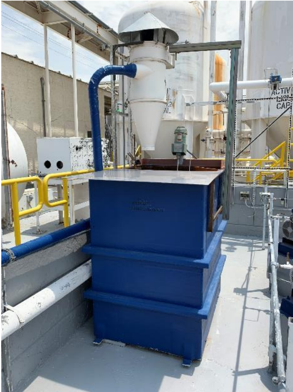
Figure 37- OU1 Scale inhibitor mixing point
