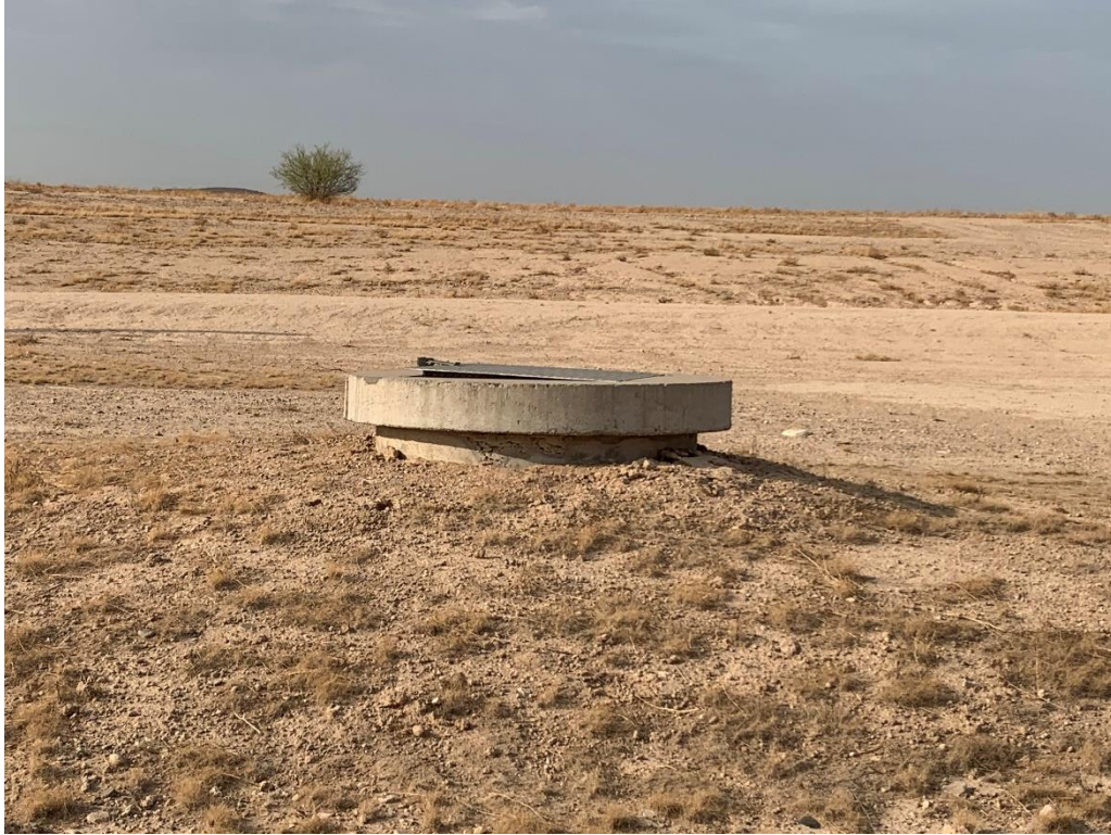
Photo 22 – Extraction well EW-2UA, showing partially closed lid
