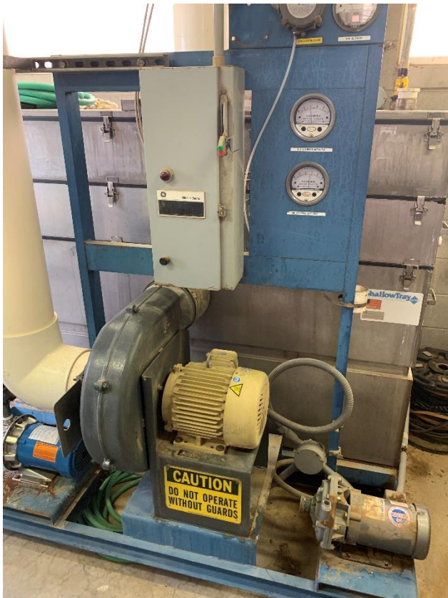
Photo 9 – Air stripper system
