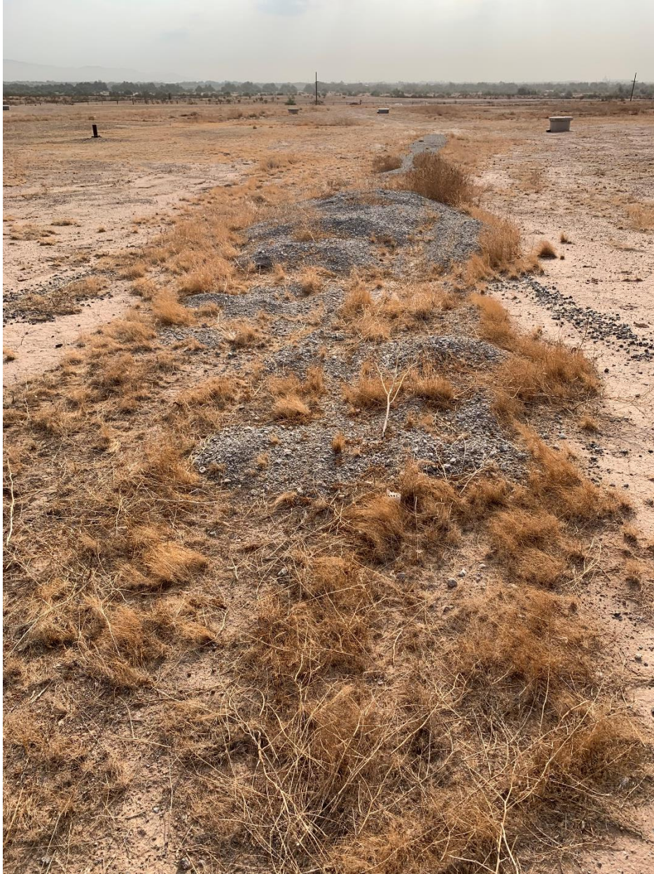
Photo 25- Gravel placed over minor erosion area, downgradient of main gate, facing east
