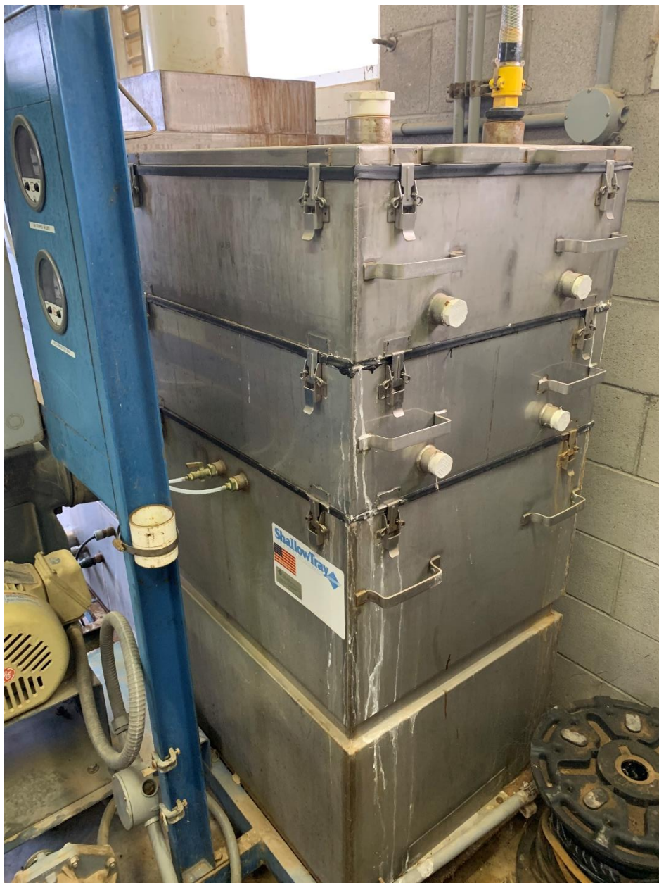
Photo 11 – Air stripper trays
