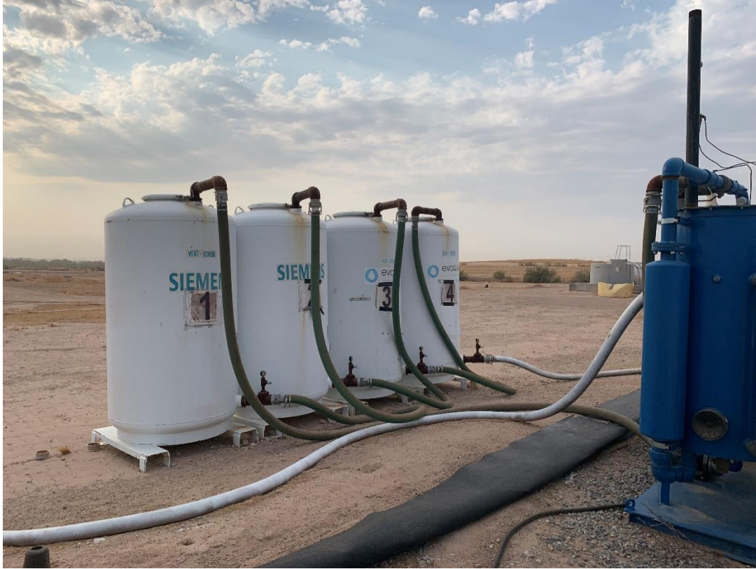
Photo 14 – View of VGAC vessels
