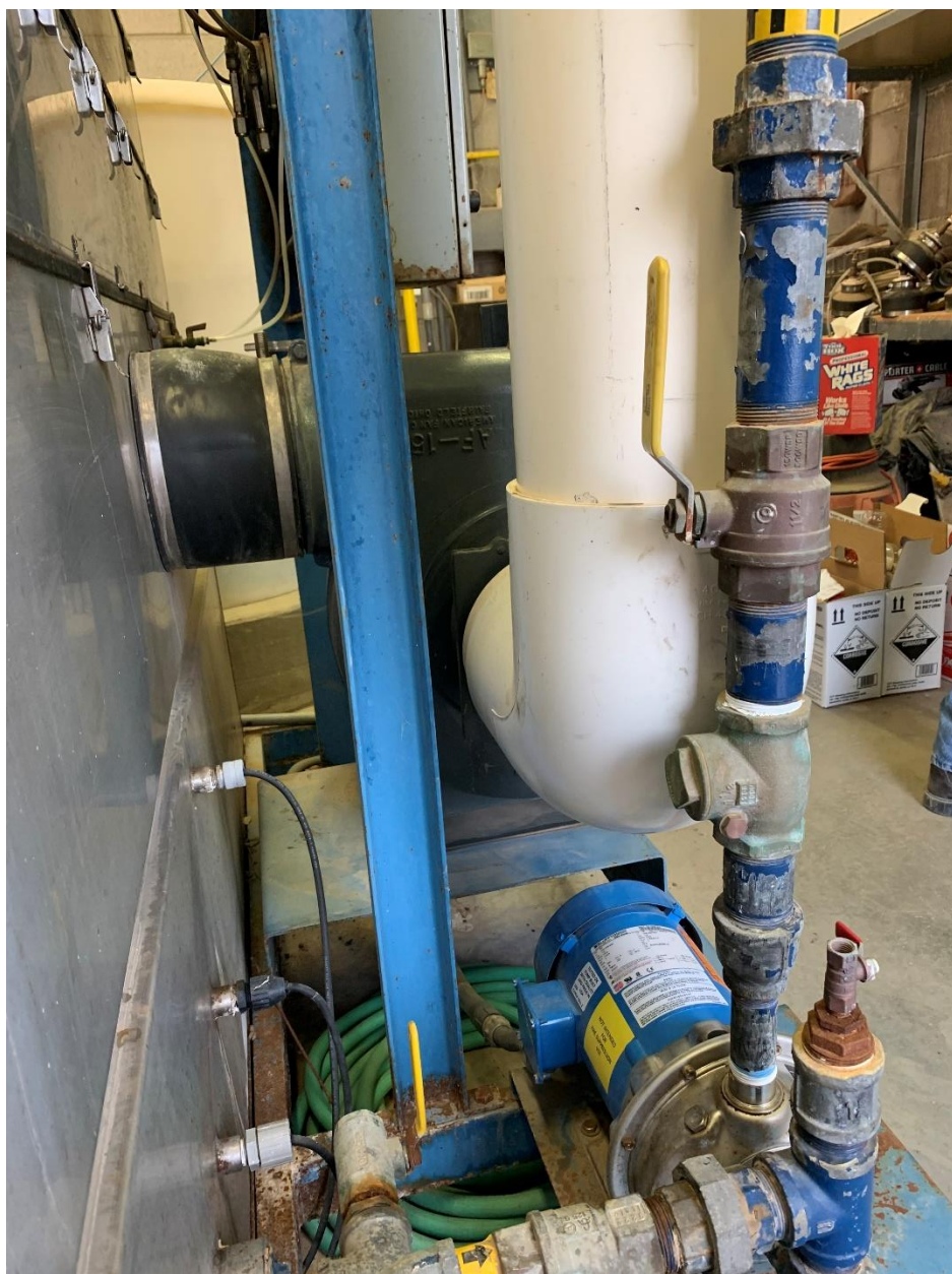
Photo 13 – View of replaced effluent check valve (center right of photo)
