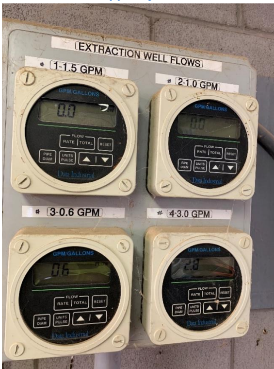
Photo 10 – Extraction well flowrate gauges
