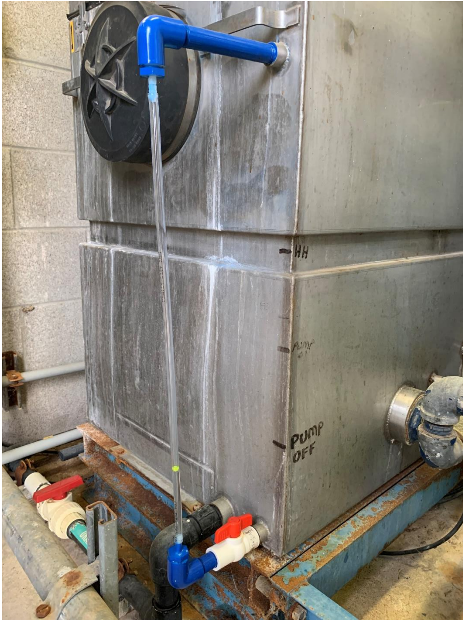
Photo 12 – Clear PVC sight glass on air stripper trays
