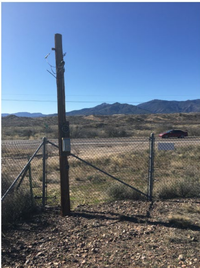
Figure 11 – Power pole and meter, disconnected
