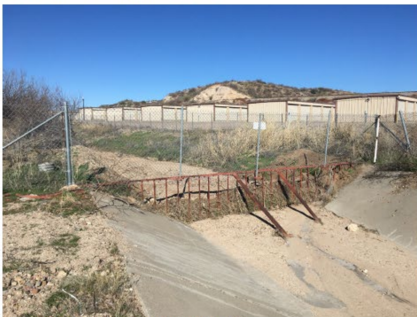
Figure 14 – Grate at upstream end of concrete channel
