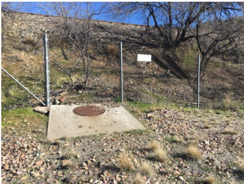
Figure 7 – Manhole for drainage channel underneath site, on north fence line
