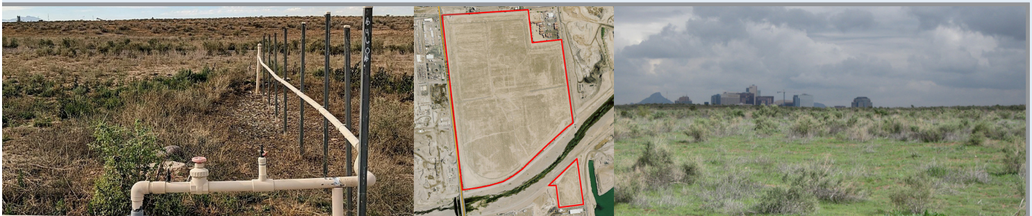
Images from left to right: View of the gas extraction system; Aerial view of the site; View of the landfill cap looking northeast toward downtown Phoenix.
