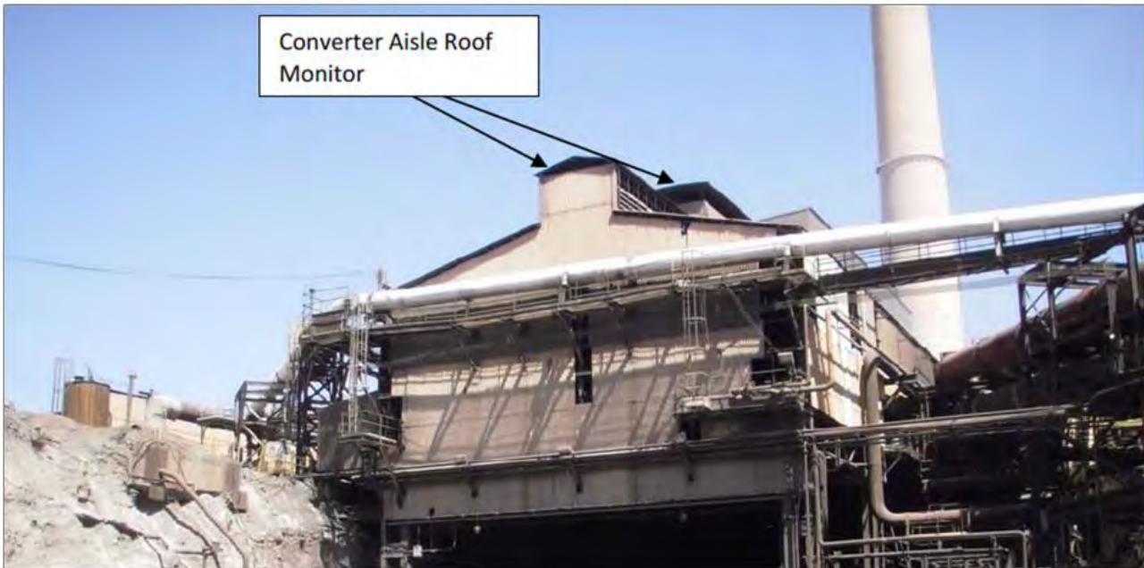
Figure 3- Converter Aisle Building Roof Monitor
