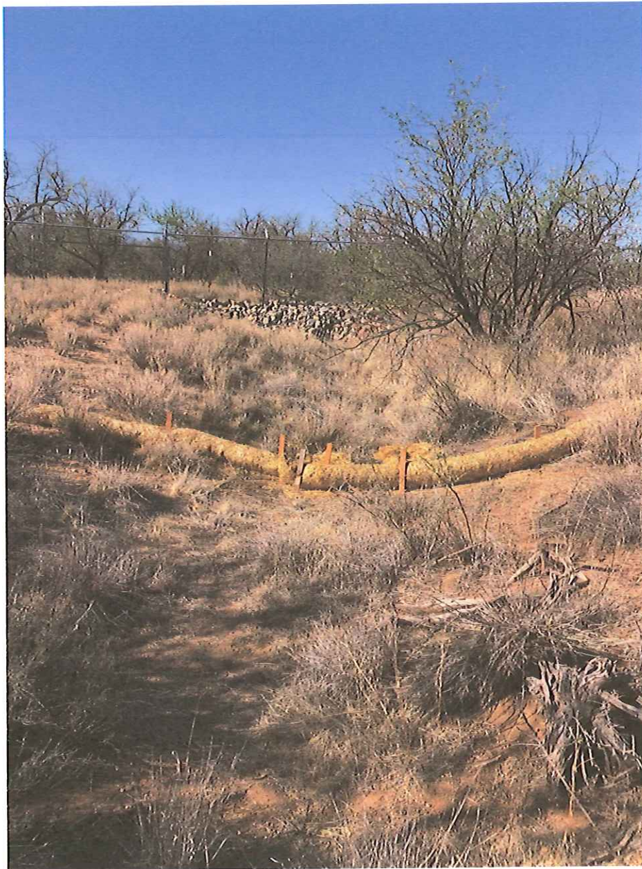
Picture 5 Installed wattle south culvert
