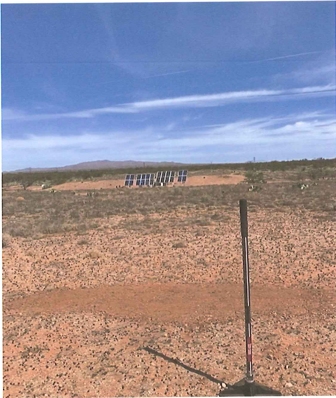
Picture 9 Repaired burrowing Cell B cover
