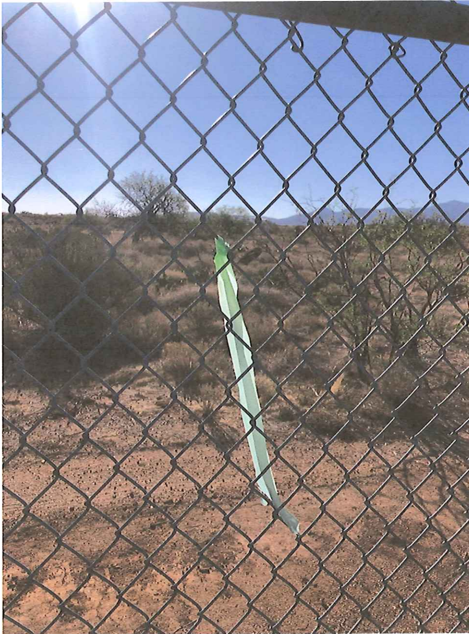
Picture 1 Location of missing sign
