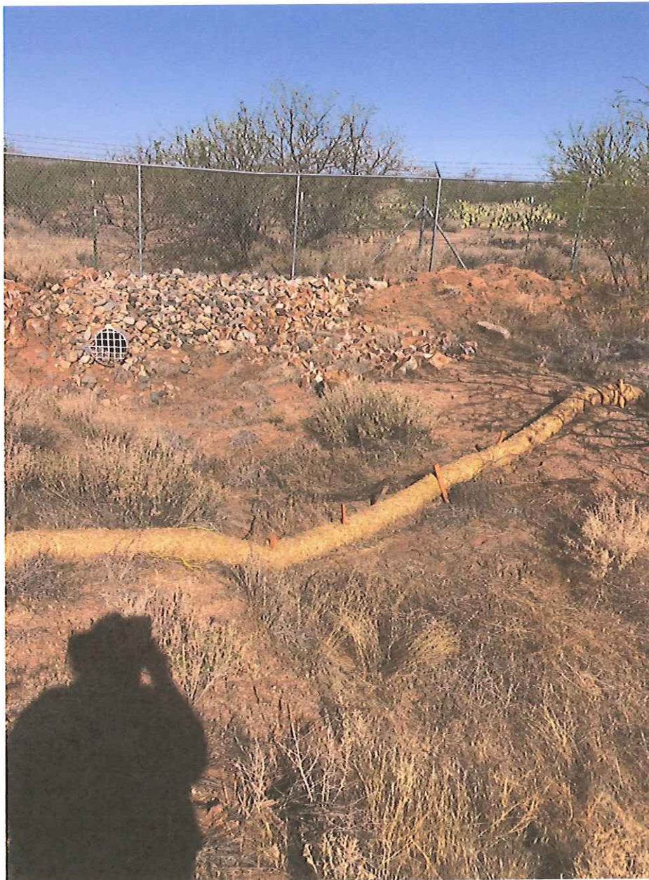
Picture 4 Installed wattle west culvert
