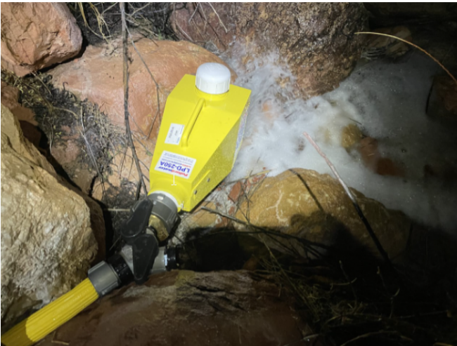
Figure 4. Discharge of effluent from Outfall 002 directly from LPD-250A dechlorinating diffuser, the final treatment process, at Phantom Ranch Delta
