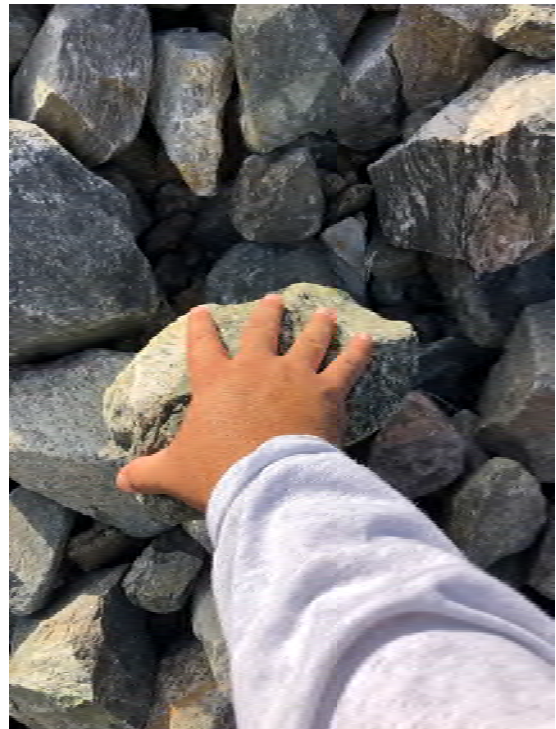
Figure 10.3 Protective Rip-rap Wall Rip-Rap Size (10-03-2018)
