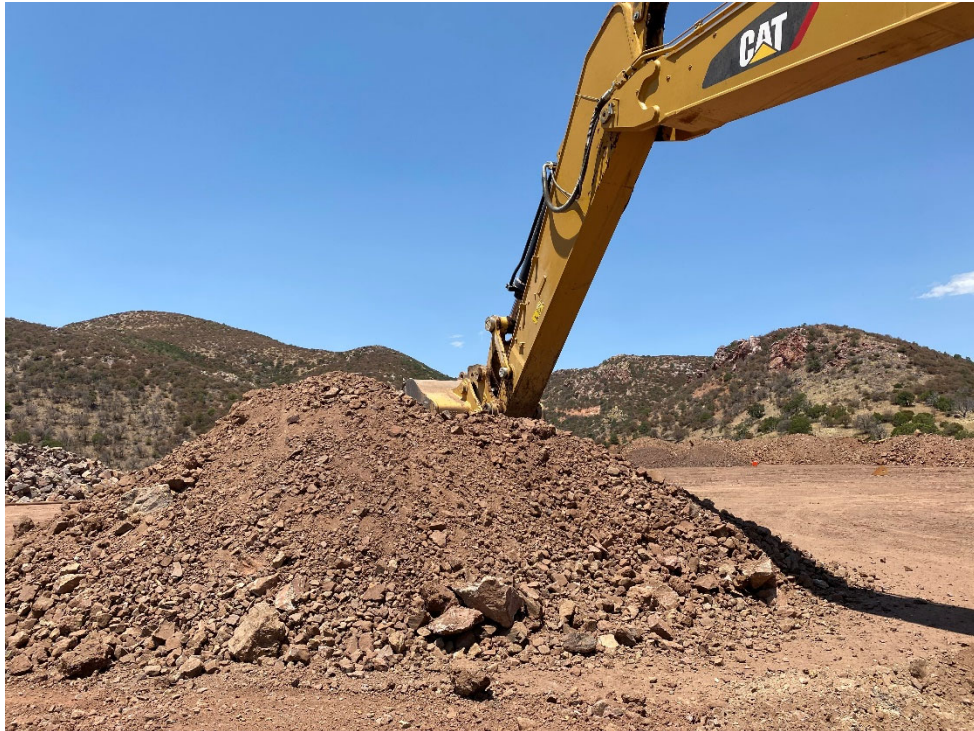
Photo 3 – TP21-19 (Existing stockpile at the IP)
