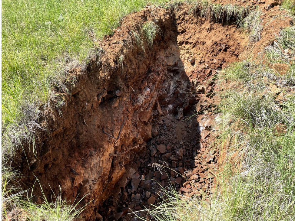
Photo 7 – TP21-03 – Shaft Platform
