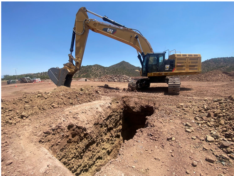
Photo 2 – TP21-22 (existing stockpile at the IP)
