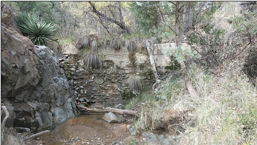
Figure 7 – Mason Dam at the Upstream End of Seep 1
