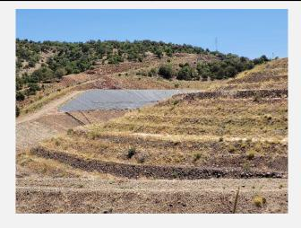
Another view of the TSF North face. Some of the TSF liner can be seen in the background. The rest of the liner is covered with tailings.
