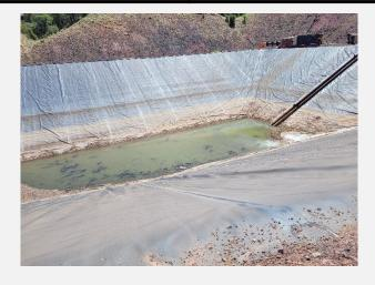
View looking East into the UCP. Minimal water can be seen at the base of the liner. The Northeast and Southwest liners were observed to be without defect.
