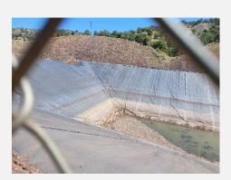
View of a dry corner of the UCP, with the Northwest embankment liner observed to be without defect or damage.
