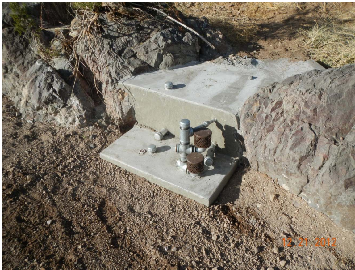
Figure 4. Float Switch Foundation (Barrel Canyon installation)
