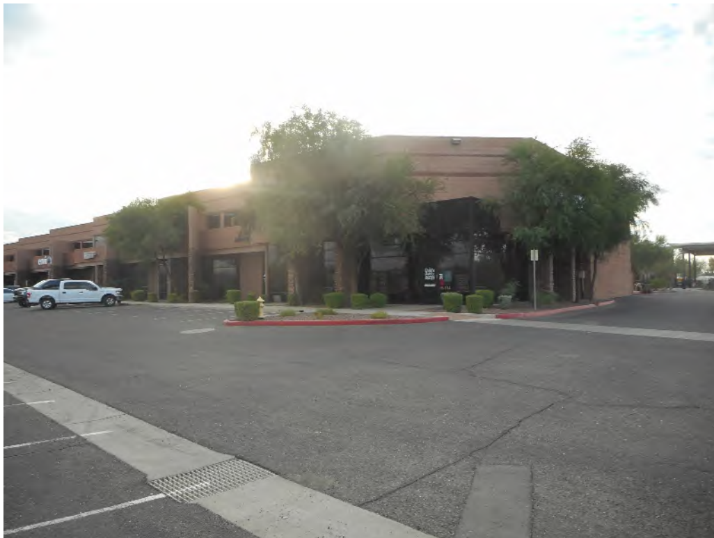
PHOTOGRAPH NO. 26 View from the northeastern portion of the Site looking east, showing the northeastern adjoining commercial buildings
