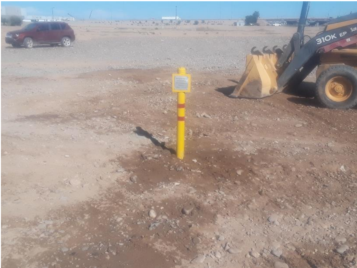
View of final site surface with well identification marker
