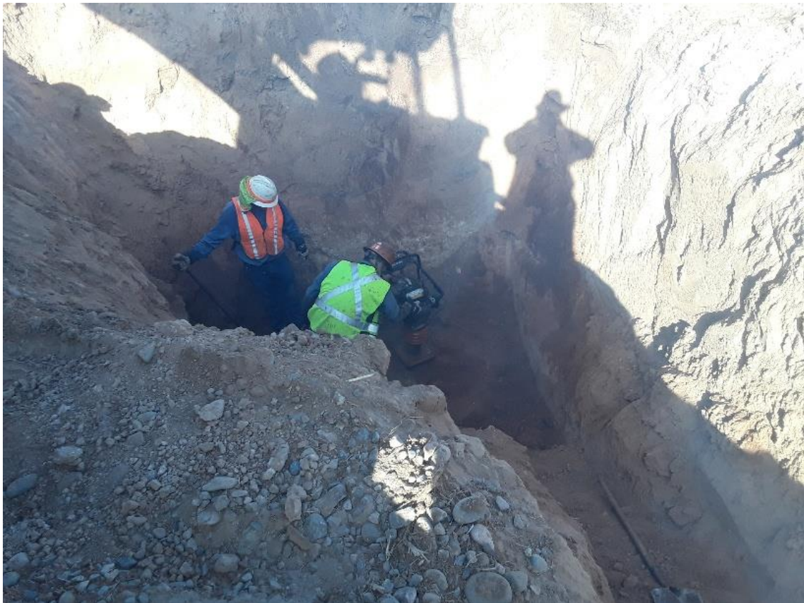
Backfill material being compacted in 1-24 excavation
