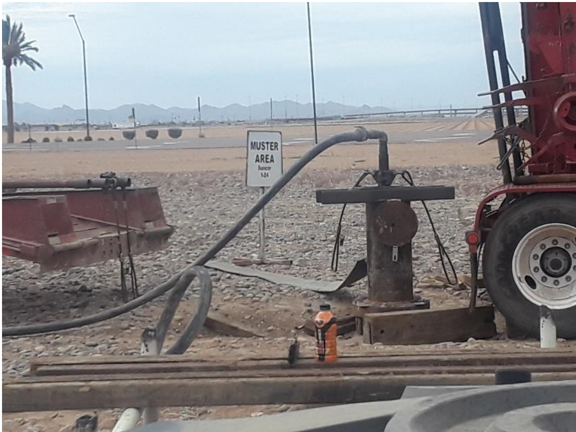
View of cement being placed down 1-24 well through tremie pipe
