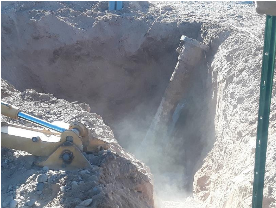
Upper 10' of 1-24 well casing being removed
