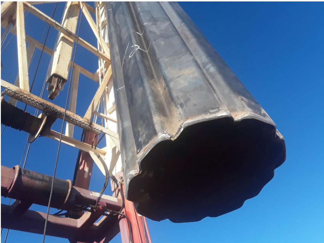
View of base of bridge plug
