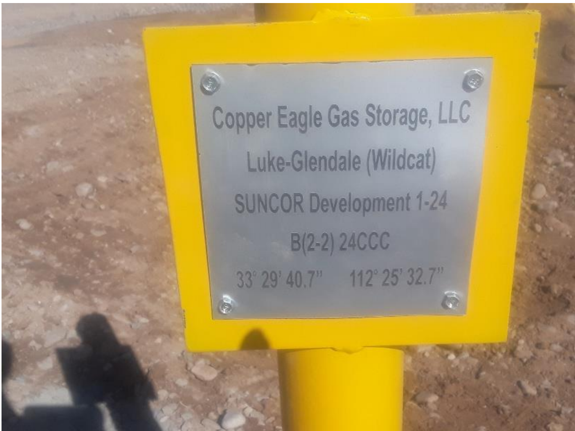
View of surface well identification marker
