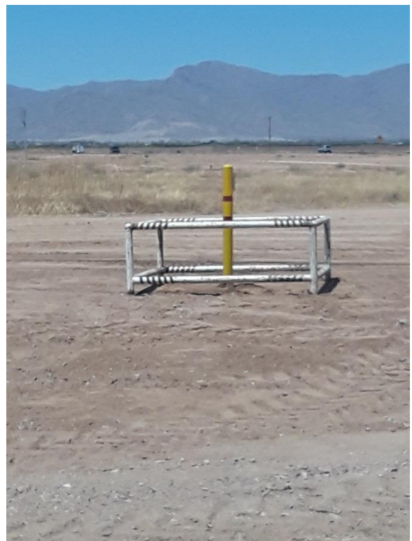
View of final site completion
