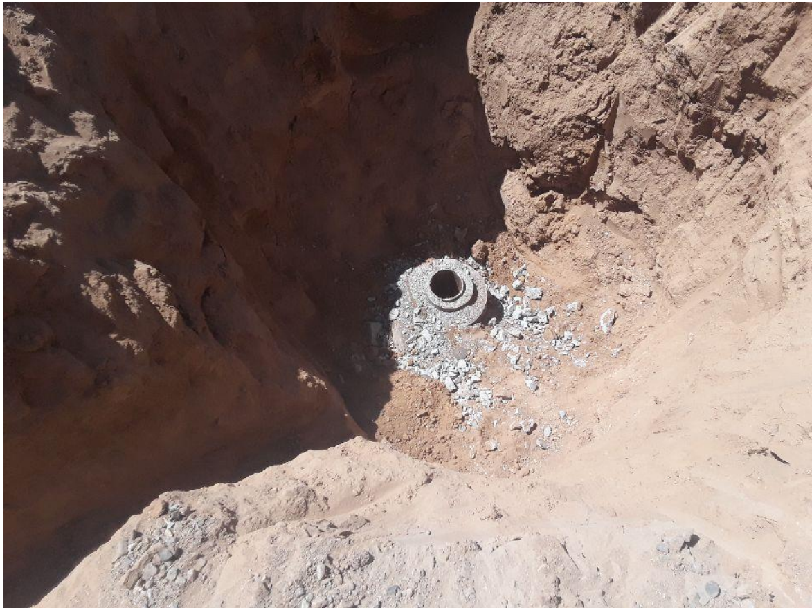
View of excavation with upper casing removed
