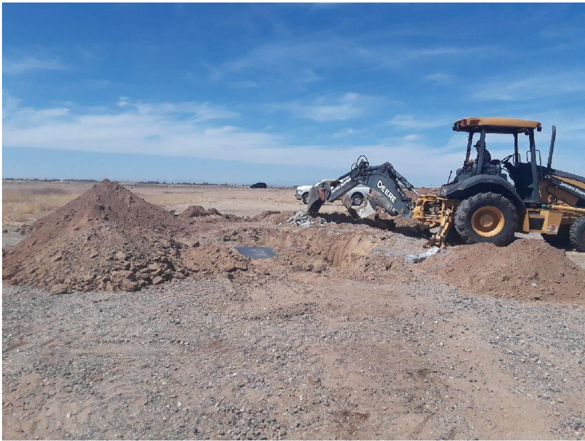
Site excavation to expose 1-19 well casing
