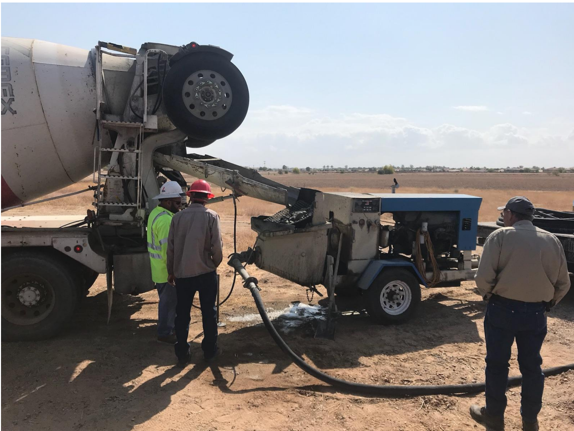
Pumping cement bentonite slurry into 1-19 well
