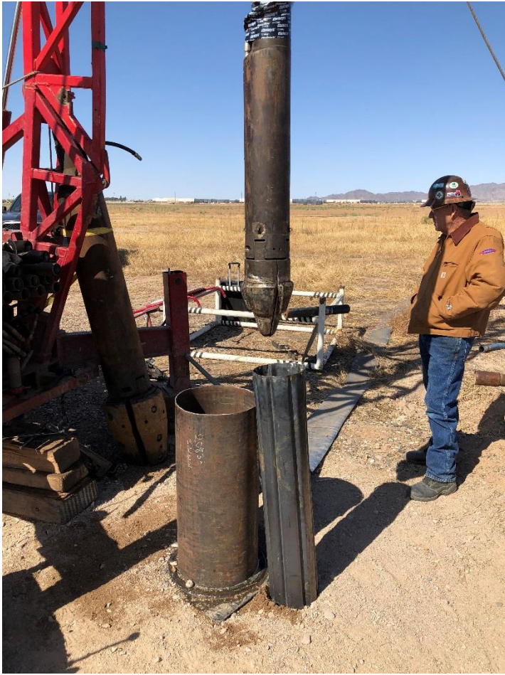
View of bridge plug and swage tool
