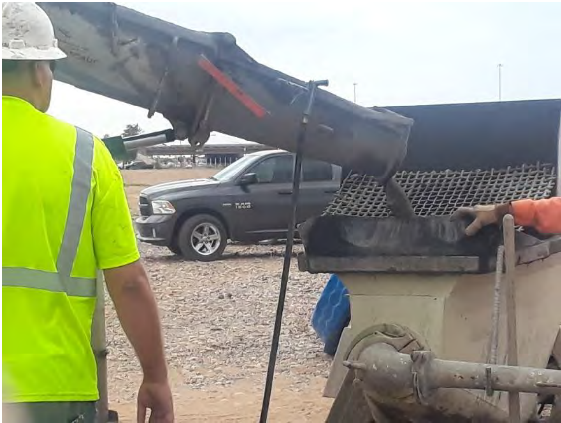
View of cement being poured into on-site strainer
