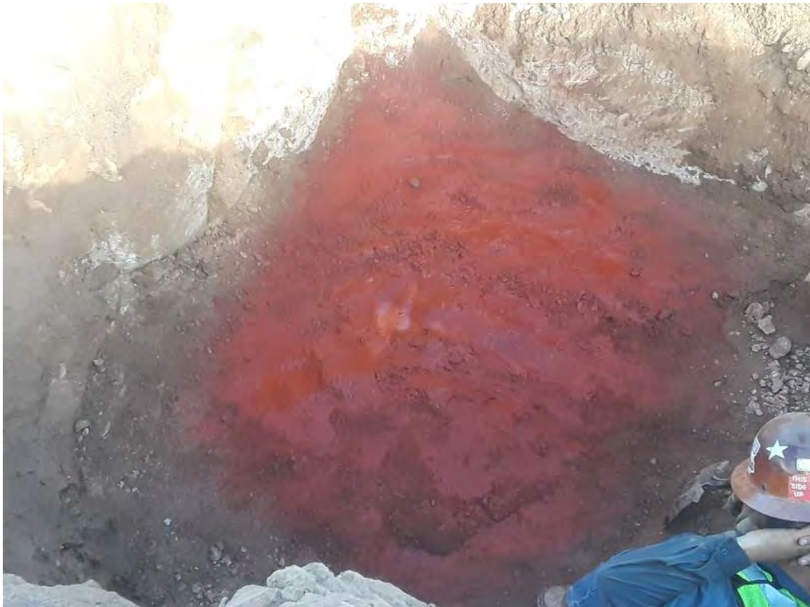
View of permanent dyed granular material over top of metal plate
