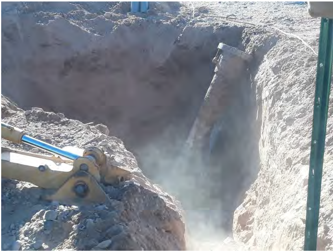
Upper 10' of 1-24 well casing being removed
