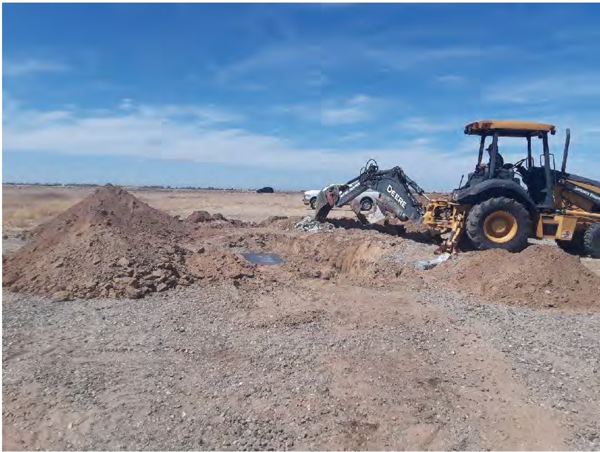
Site excavation to expose 1-19 well casing
