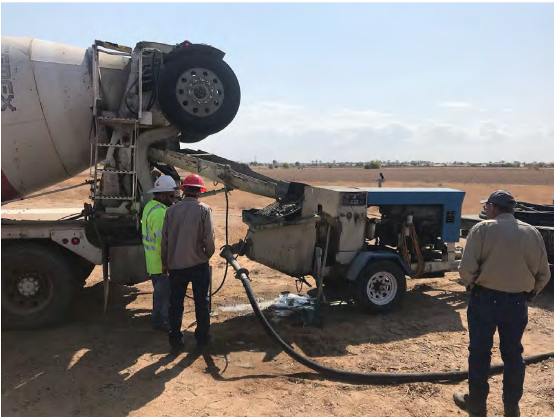
Pumping cement bentonite slurry into 1-19 well
