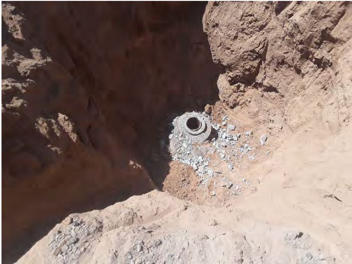
View of excavation with upper casing removed
