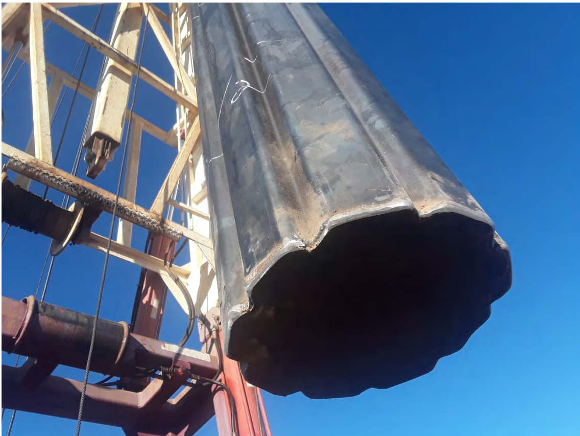
View of base of bridge plug
