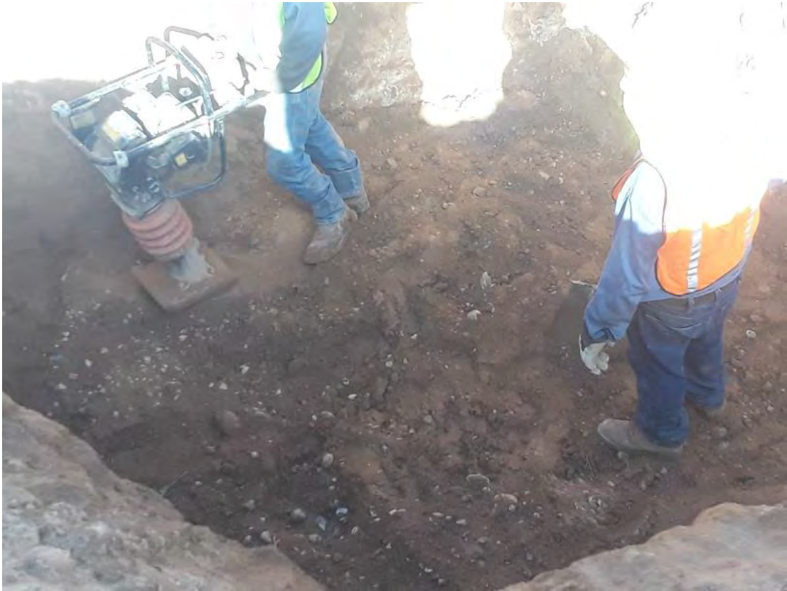
View of imported fill material being compacted in excavation
