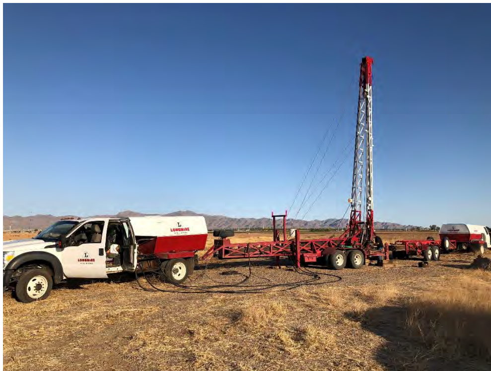
View of Longmire rig
