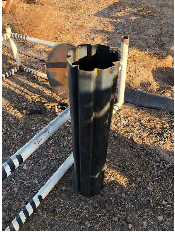
View of bridge plug
