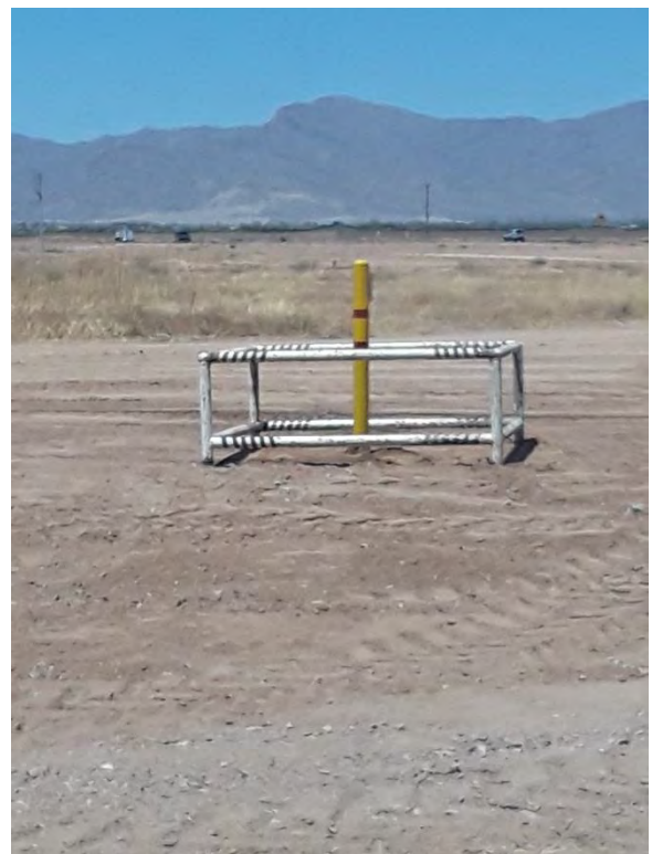
View of final site completion
