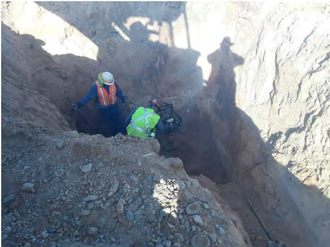
Backfill material being compacted in 1-24 excavation
