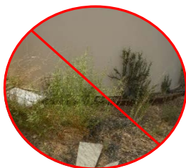
Excessive vegetation around storage tank
