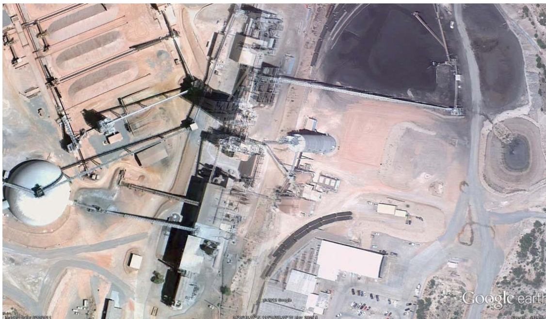
Figure 5. Phoenix Cement Plant, Clarkdale, AZ
