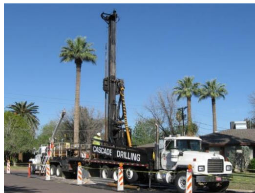
Groundwater Monitoring Well Installation
