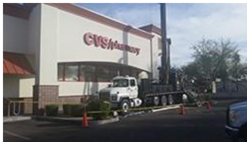
Drilling of Groundwater Monitoring Well at CVS Pharmacy
