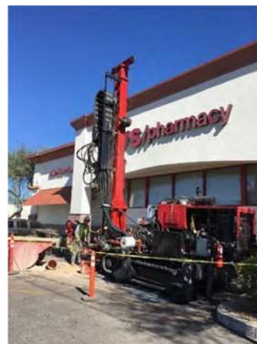
Drilling of Soil Vapor Monitoring Wells at CVS Pharmacy
