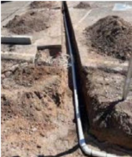
Continued operation of the SVE system including in-situ treatment of the soil; decommissioned groundwater extraction treatment system
