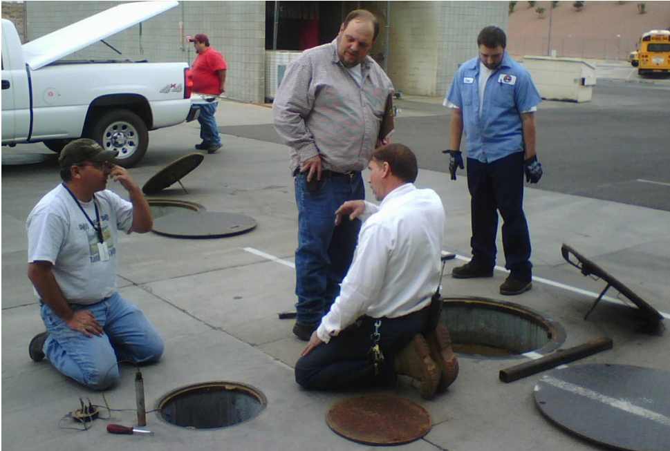
ADEQ Inspectors demonstrate a routine UST Inspection to UST operators.
